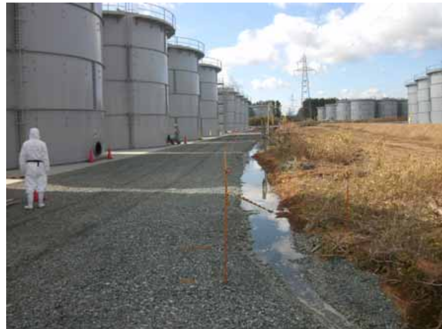
Photo taken on March 26, 2012 by TEPCO
