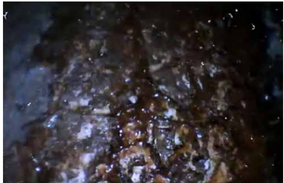
Floor surface where the water leakage could have occurred
