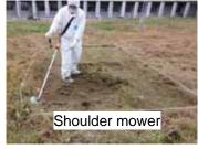
Stripping the turf surface with a mower
