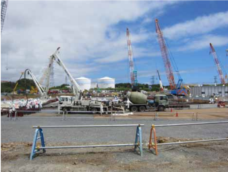
-1 Multi-nuclide Removal Facility construction site (Full-view) Photo taken by a TEPCO employee on June 11, 2012
