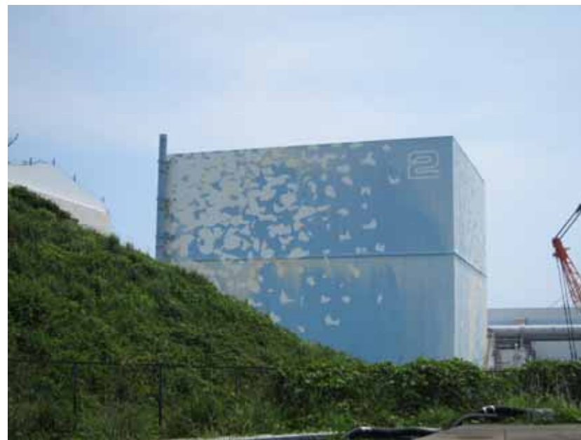
-2 Appearance of Unit 2
