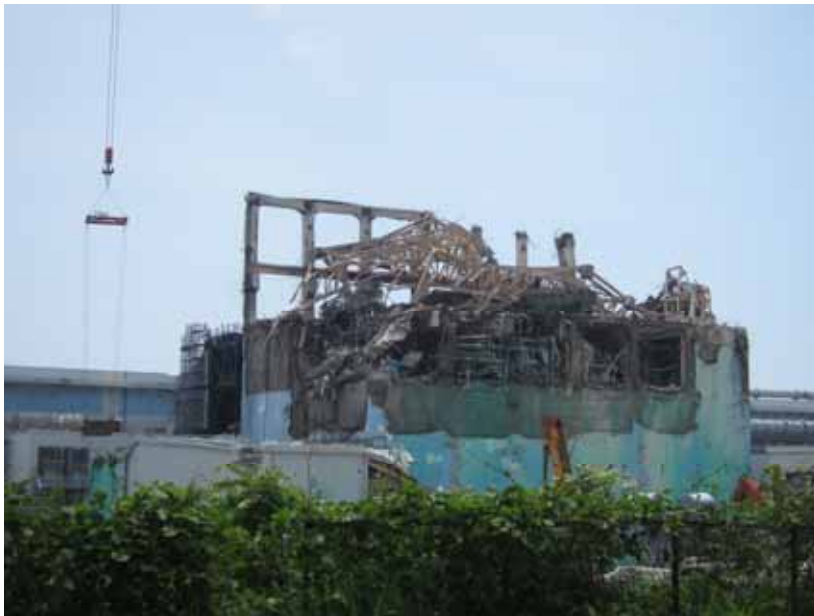
-3 Upper part of Unit 3 Reactor Building Photo taken by a TEPCO employee on June 18, 2012
