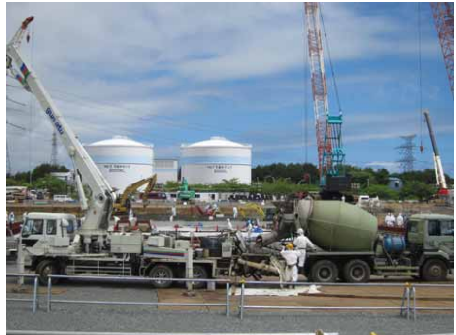
-2 Multi-nuclide Removal Facility construction site (Full-view): Foundation improvement work Photo taken by a TEPCO employee on June 11, 2012
