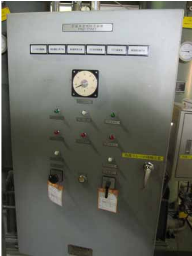
Control panel of the compressed air system (IA system)
