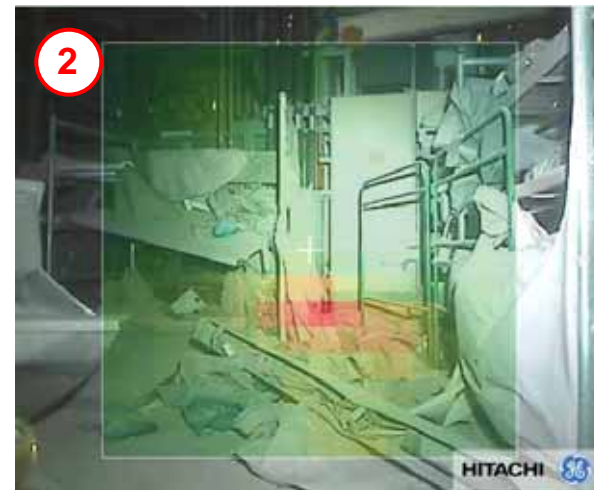
Image acquired at the northwest corner before BG correction (Angle of elevation: 0 degrees)
