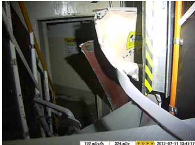
In front of Southwest stairway
