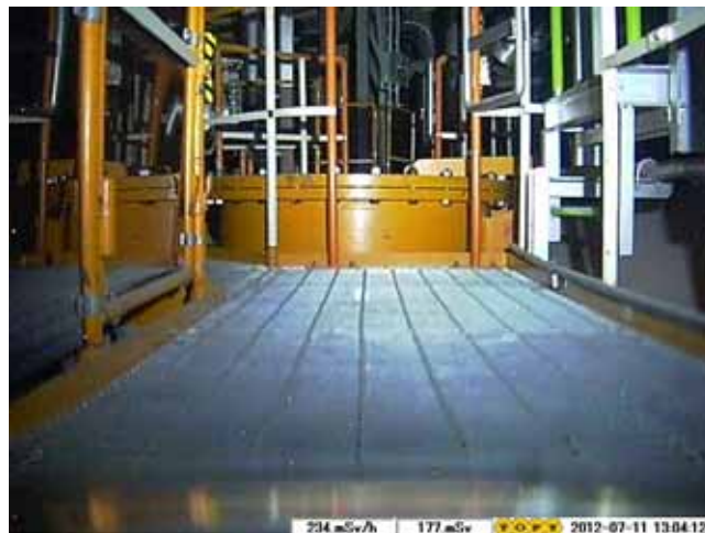
Southeast side manhole
