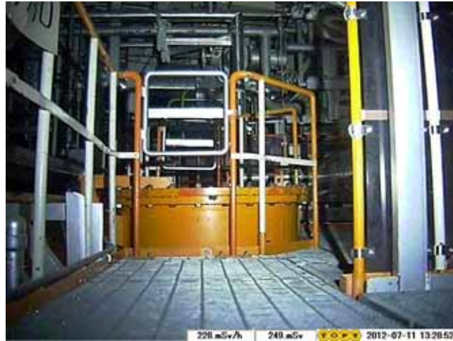
North side manhole
