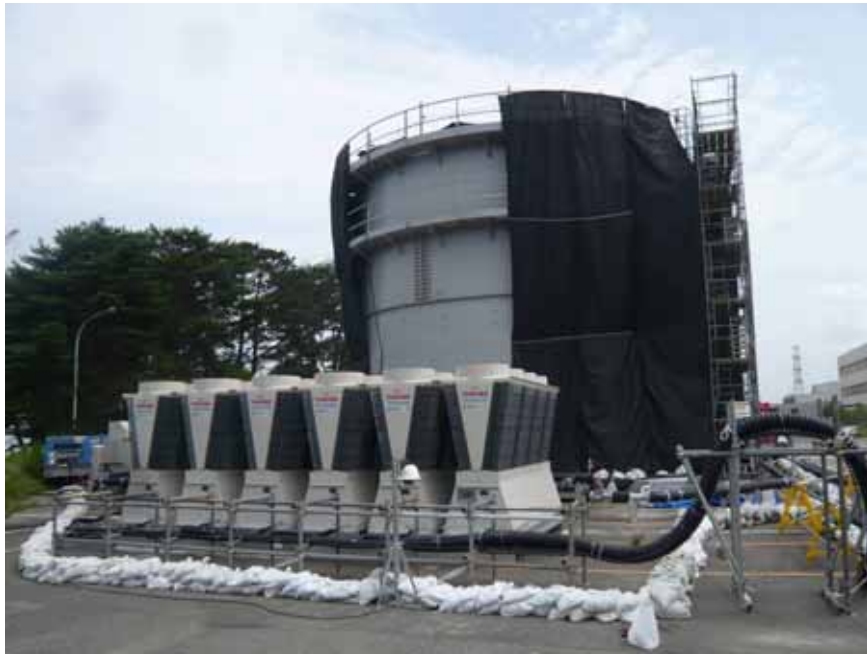
Back: Treatment water buffer tank, Front: Refrigerators Photo taken on July 13, 2012
