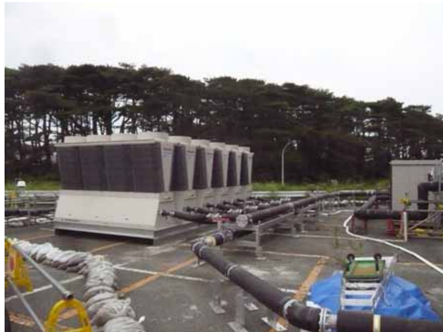
Pipe connection for the refrigerators Photo taken on July 13, 2012
