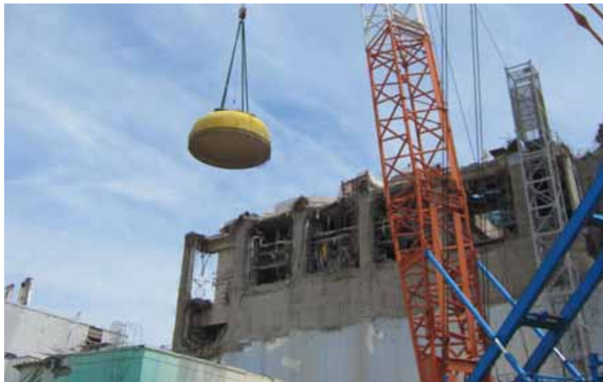
PCV upper lid being lifted up in the upper part of the operating floor
