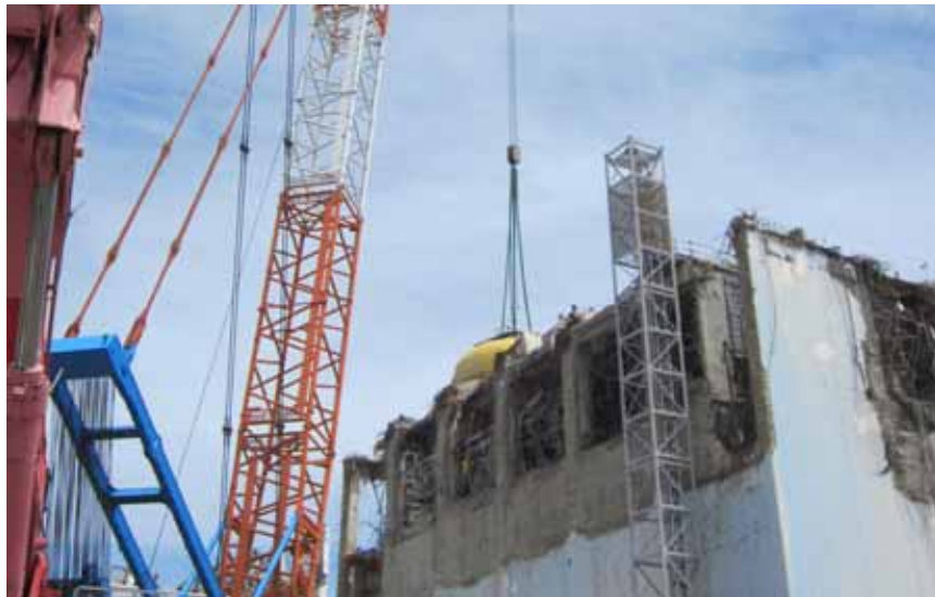
PCV upper lid on the upper part of the operating floor
