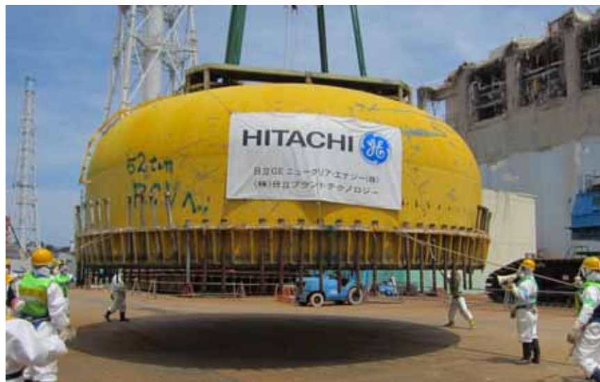
PCV upper lid being lifted down to the ground (2)
