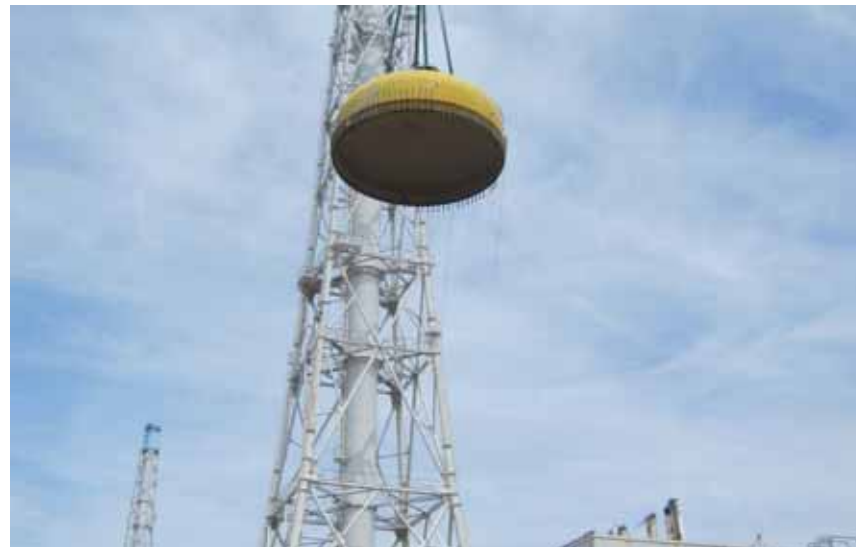
PCV upper lid being lifted down to the ground (1)
