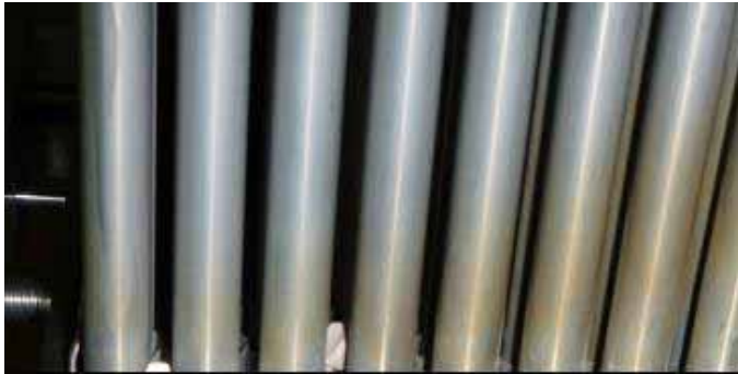
1. First unused fuel (Rust attached on the surface) (Photo taken on August 28, 2012)
