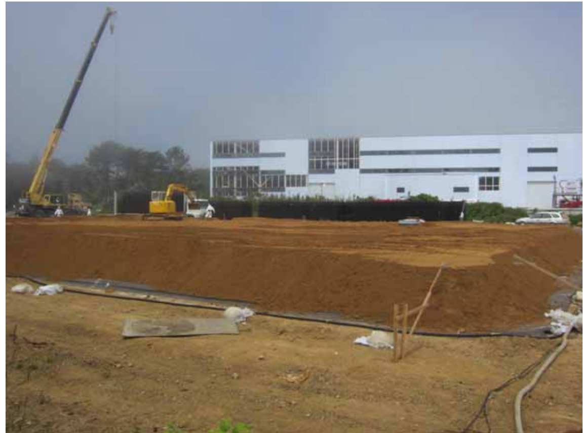
-2 Underground water storage tank installation
