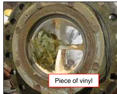
The back side of the suction part (Photo taken from the back side after removing the suction part from the pump)
