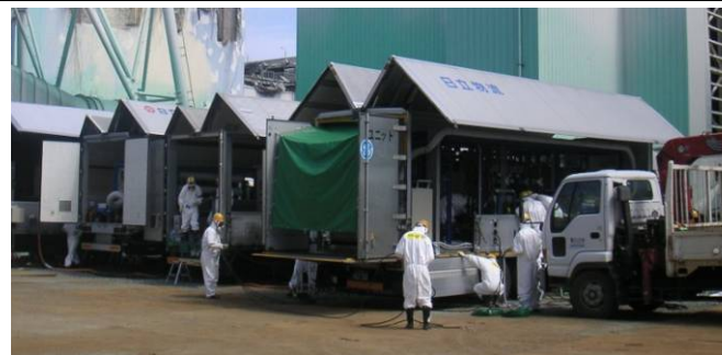
Reverse osmosis membrane (RO) system used for desalting
