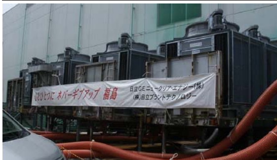
Circulation cooling equipment for the spent fuel pool
