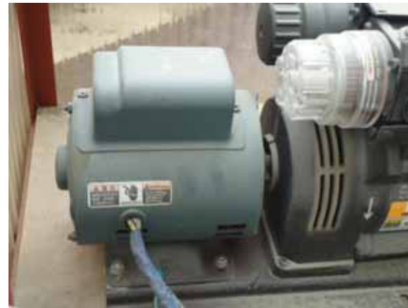
Appearance after the smoke stopped coming out (October 2)
