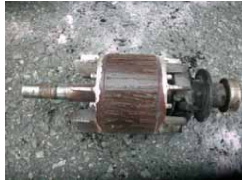
Inside the electric motor of G pump (rotor)
