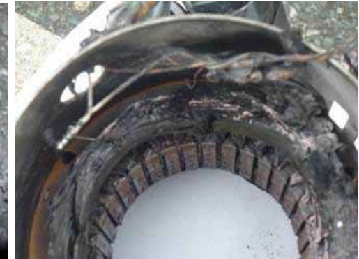
Inside the electric motor of G pump (stator)
