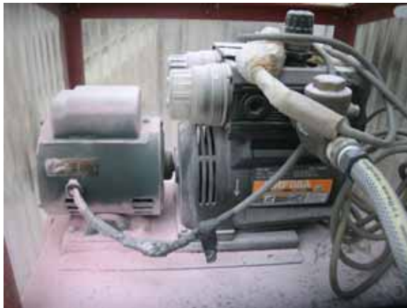
Appearance after the smoke stopped coming out (August 14)
