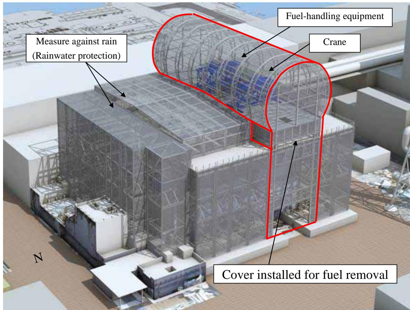
Cover installation for fuel removal at Unit 3 (Northwest side)
