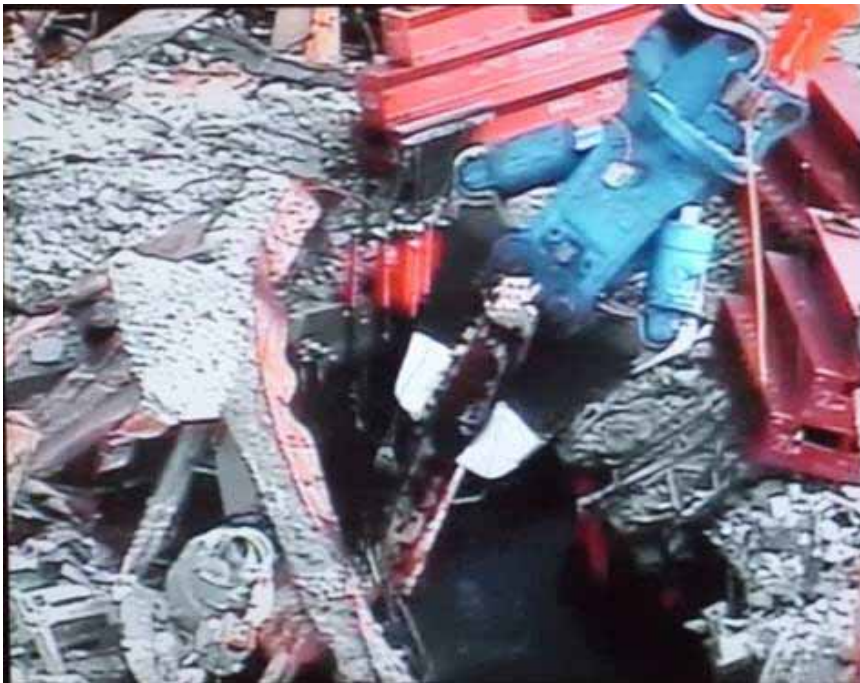
Steel beam which fell into the pool (When being lifted)
