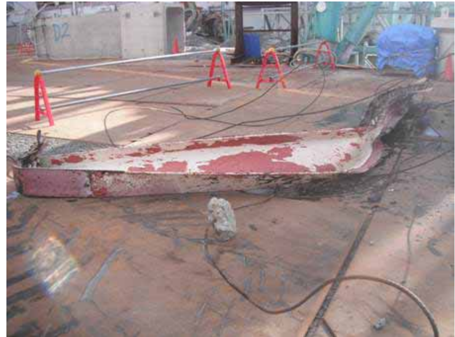
Steel beam which fell into the pool (After being removed)
