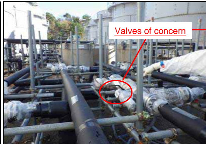
[Area surrounding the leakage location]
