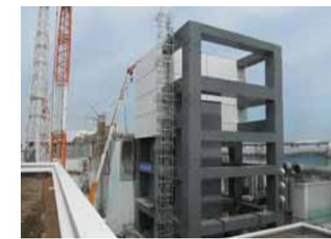
Progress of steel frame construction (Photo taken on April 23)
