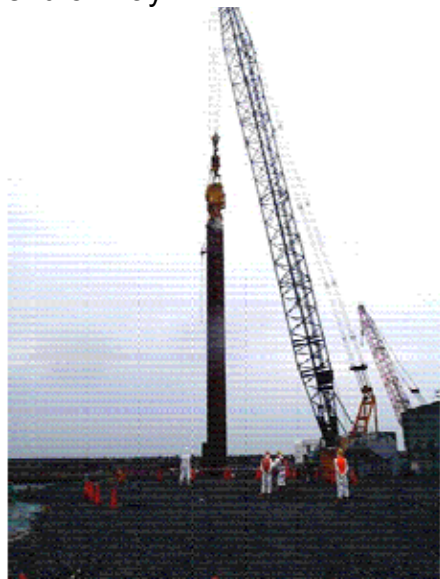
2. Installation of steel pipe sheet piles for impermeable walls
