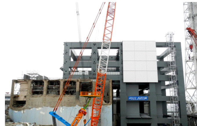
The steel frame was completed (Photo taken on May 29)
