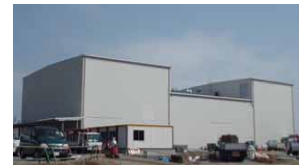
Figure 5: Exterior appearance of the entrance control facilities
