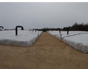
Temporary trimmed trees storage pool
