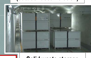
Solid waste storage
