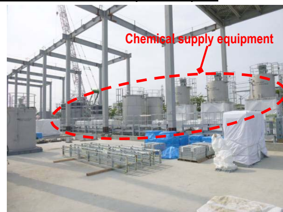
Figure 3: Installation status of additional multi-nuclide removal equipment
