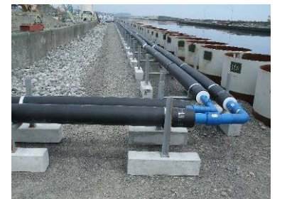
Installation status of groundwater drain pipes
