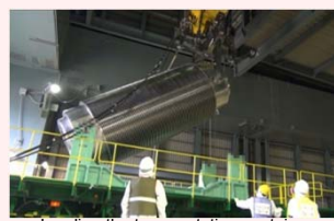
Loading the transportation container onto the trailer
