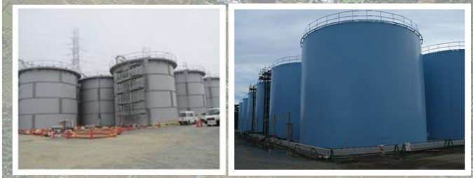
Tank installation status
