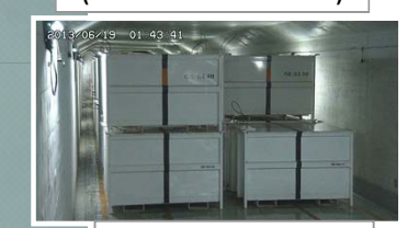
Solid waste storage
