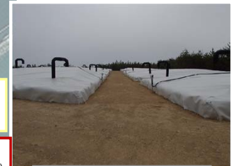
Temporary trimmed trees storage pool
