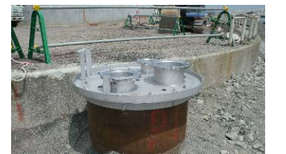
Installation status of groundwater drain pumping well (in front of Unit 1 intake)
