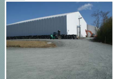
Rubble storage tent
