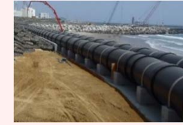
Water pipe installation status (2)
