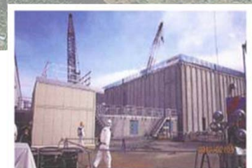
Temporary waste sludge storage
