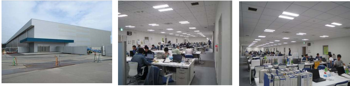
Figure 14: External appearance and work at the new Administration Office Building
