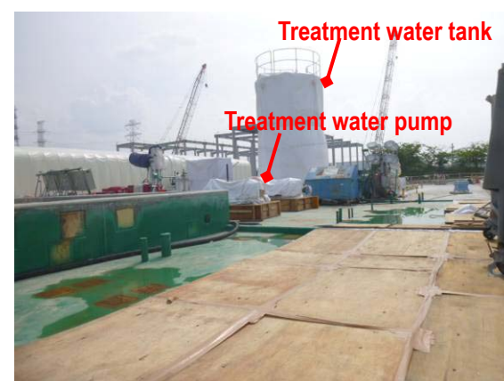
Figure 4: Installation status of high-performance multi-nuclide removal equipment
