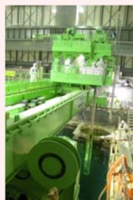
Fuel removal status
