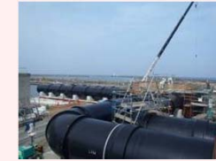
Water pipe installation status (1)
