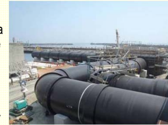
<Installation status of water pipes>
