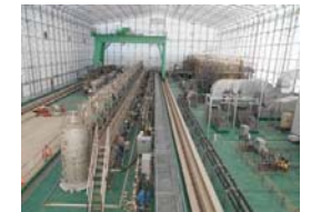
(Installation status of high-performance multi-nuclide removal equipment)
