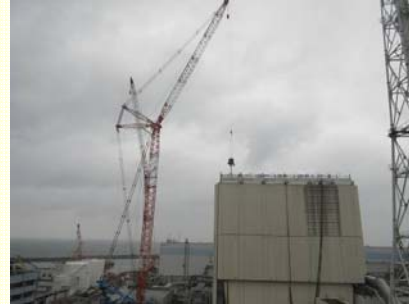
<Opening of roof panel holes and spraying of anti-scattering agents>
