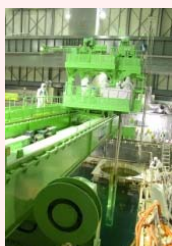
Fuel removal status
