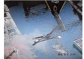
(Mar 6: Removal of fuel-handling machine west-side frame)
