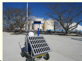
< Installation of Dose-rate monitor >
