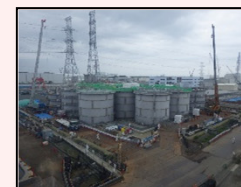
When dismantling started
