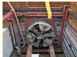
< Construction of tunnel part to switch K drainage channel >
