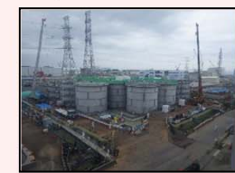
When dismantling started
