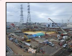
After dismantling in H1 east area
