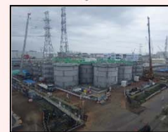
Start of dismantling in H1 east area
