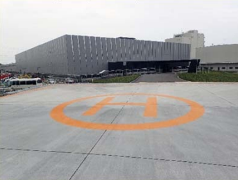
<Heliport (near the Main Administration Building)>
