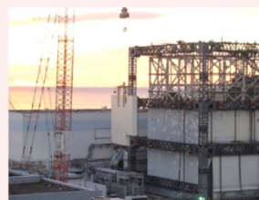
<Dismantling of wall panels>
