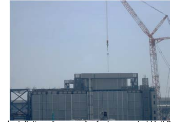
Installation of a cover for fuel removal at Unit 3 (May 22, 2017)
