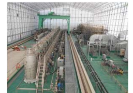
(High-performance multi-nuclide removal equipment)
