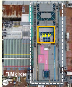
<After installation of the FHM girder>
