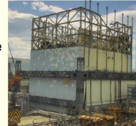
<After removal of pillars and beams>
