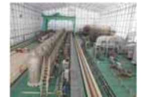
(High-performance multi-nuclide removal equipment)
