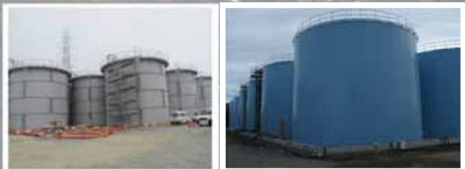
Tank installation status
