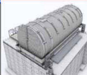
Image of the cover for fuel removal
