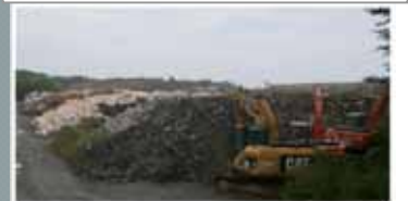
Rubble (outdoor accumulation)
