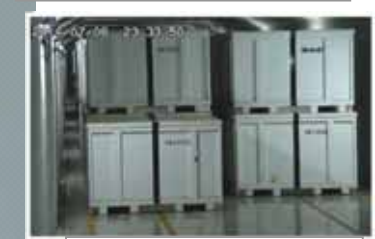
Solid waste storage facility
