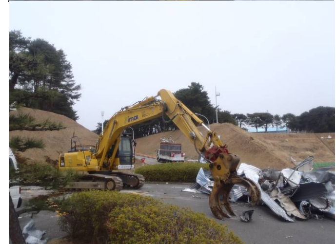
Debris on the ground
