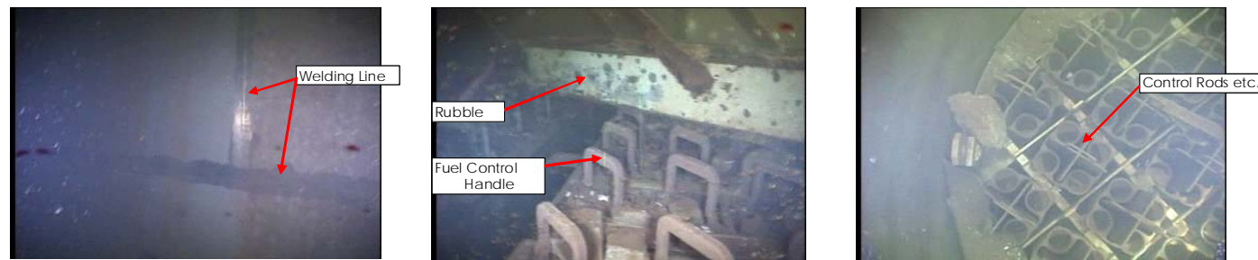
① Southern Wall Surface ② Rubble and Upper Part of Spent Fuels ③ Cask Pit Inside
