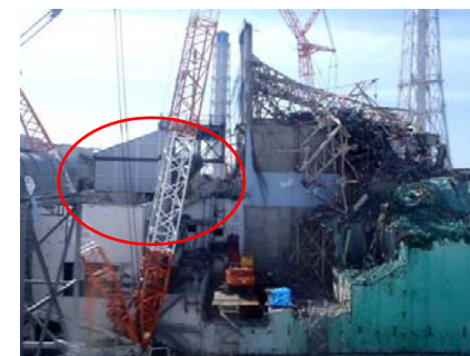
Unit 3 Reactor Building Installed a gantry for upper rubble clearing (eastside)
