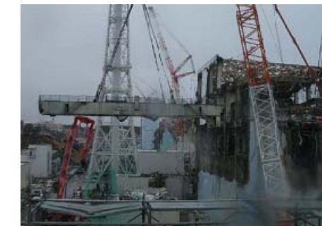
Unit 4 Reactor Building Removing Overhead Crane Garter
