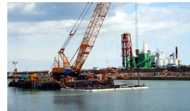
Fig. 3: Implementing Seabed Covering Work in front of the Units 1~4's Intake
