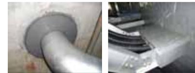
Example of waterproof treatment at pipes and cables
