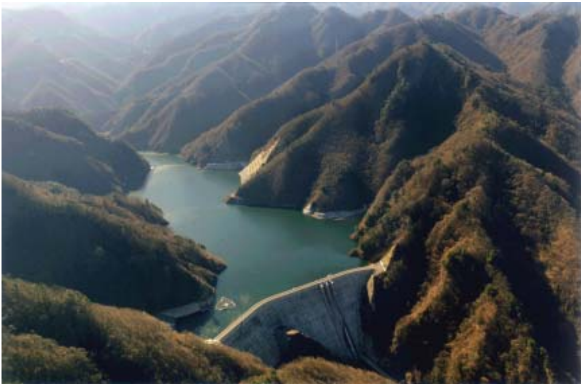
Ueno Dam (lower dam) of Kannagawa Power Plant
