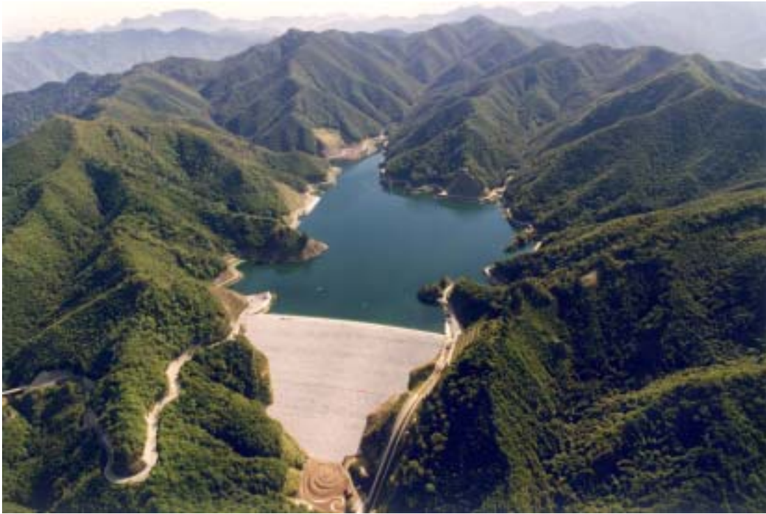
Minamiaiki Dam (upper dam) of Kannagawa Power Plant
