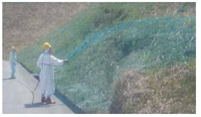
Dispersion of inhibitors in the Power Station (slope)
