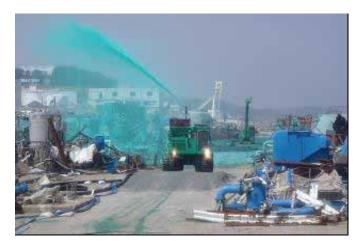
Dispersion of inhibitors around turbine buildings of Units 1 to 4
