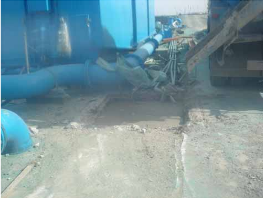
Concrete placement case
