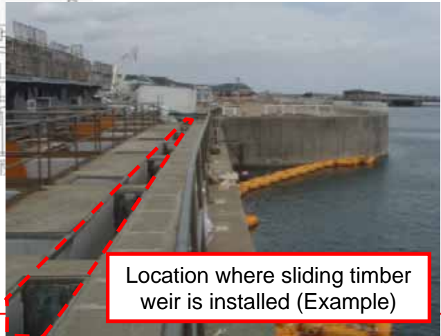
Sliding timber weir in seawater pump house for auxiliary equipment cooling was already installed.
