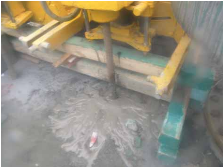
LW (liquid glass + mortar) injection case
