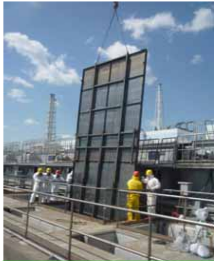
Steel plates were already installed (Unit 2) (completed by April 15)
