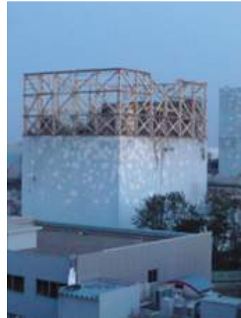
Explosion of Unit 1 Reactor Building
