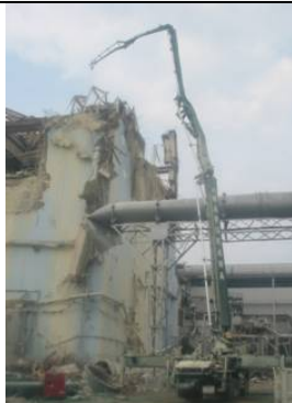
Sampling by concrete pumper
