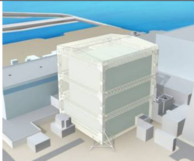
Installation Image of the Unit 1 Reactor Building Cover
