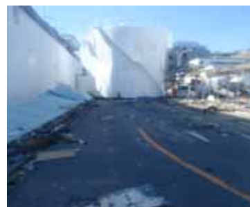
Tank washed up by tsunami
