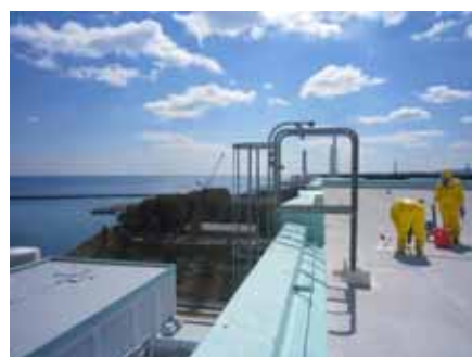
Work conditions on the roof
