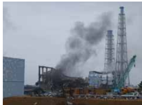
Unit 3 after explosion
