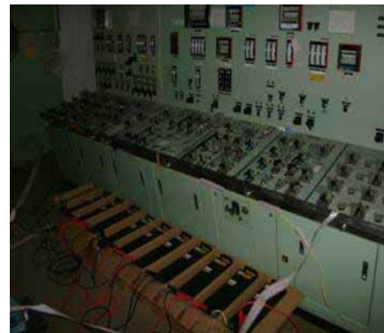
Connecting temporary battery to power instrumentation
