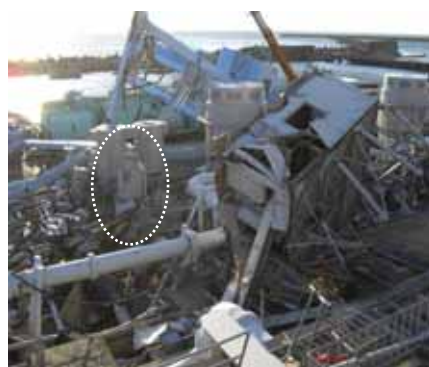
Condition of seawater pump area ( : indicates the DG (6A) seawater pump)
