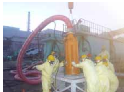
Work conditions for installation of underwater pump
