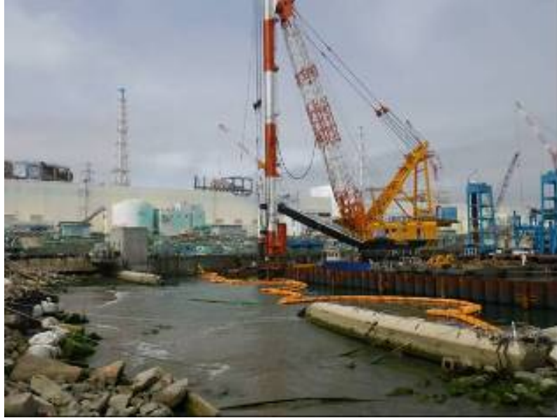
Status of placing steel pipe sheet pile
