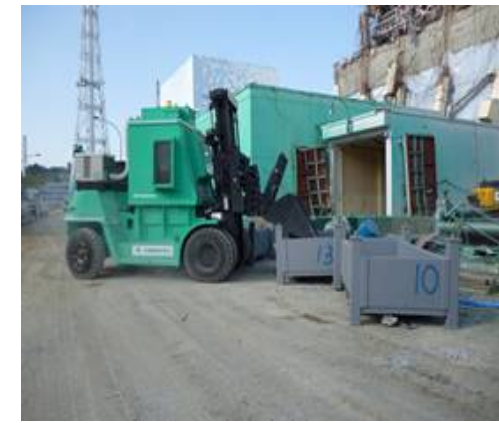
Container loading using shielded forklift
