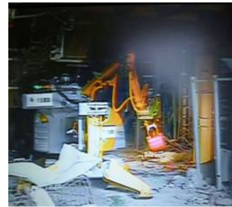
Removal of debris using Brokk (wired remote control)
