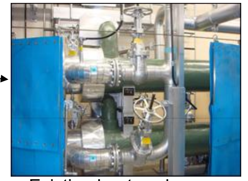
Existing heat exchanger
