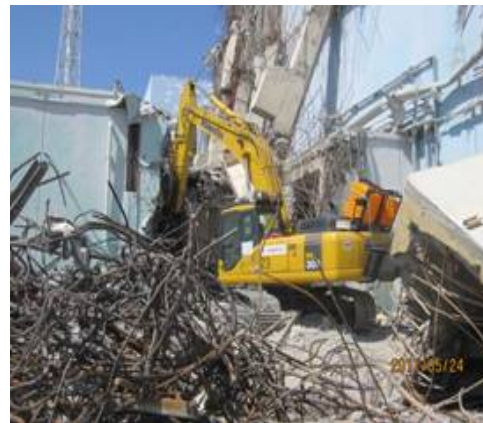
Removal of outside pillars using wirelessly-controlled backhoe
