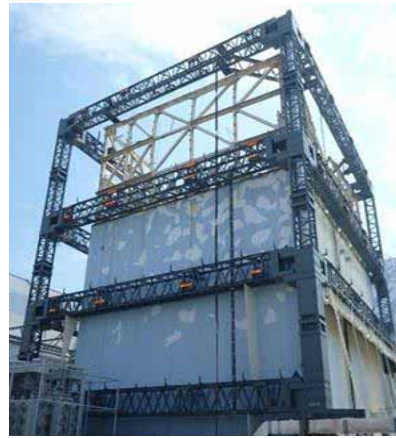
Completion of steel framing
