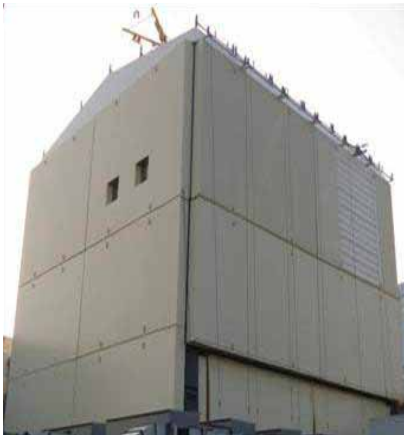
The Covering was completed
