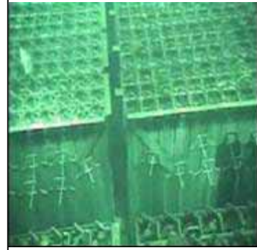
Inside the Unit 4's Spent Fuel Pool
