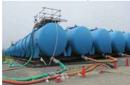
Concentrated waste liquid tank
