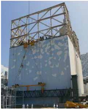
Start of steel framing
