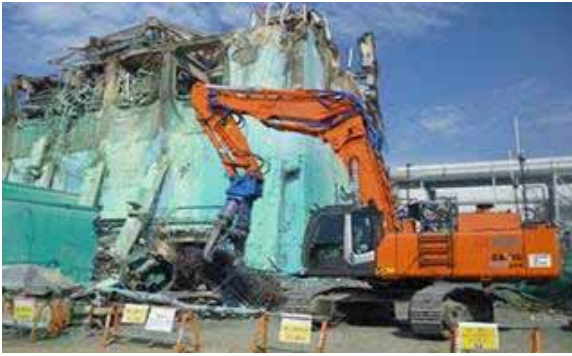
Removal of the debris fallen around Unit 3 R/B
