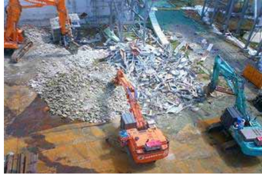
Demolition of the obstacles around Unit 4
