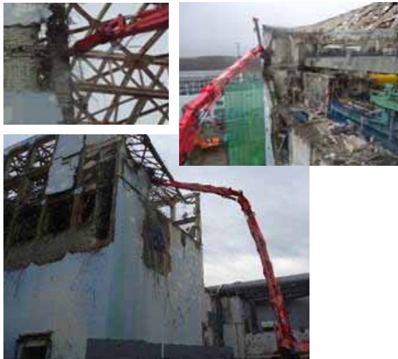
Debris removal at the top
