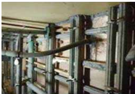
Injecting grout (Jul. 30)
