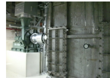
SGTS •No external equipment abnormality A/B alternating operation
