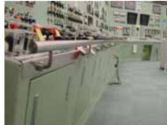
Installation of a handrail at the control panels in the Main Control Room
