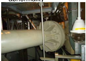
Stabilizer (in PCV) •No external equipment abnormality
