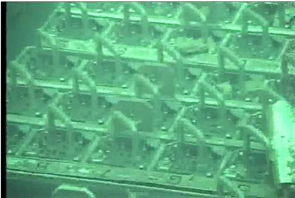
Figure 9 Conditions within Unit 4 SFP (4)
