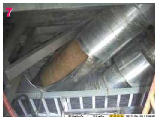
7 South corridor upper area
