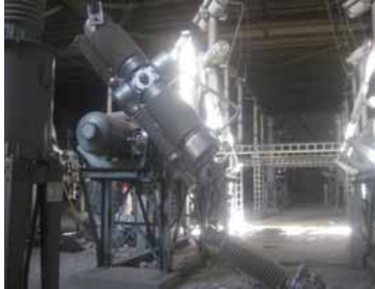
Figure 1. Fukushima Daiichi Nuclear Power Station Okuma 1L circuit breaker
