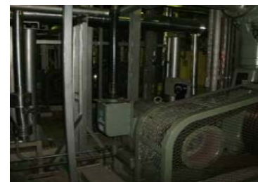
Instrumentation air compressor •No external equipment abnormality
