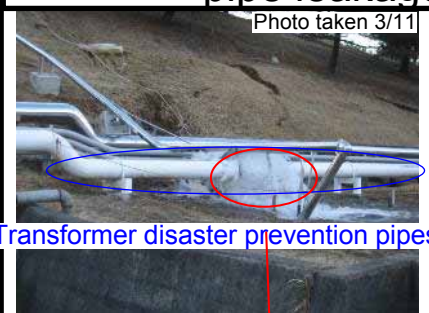
• Support for another pipe at a joint for the transformer disaster prevention pipe (filtered water tank source) became slanted due to collapse of the slope. Said joint made contact and caused leakage.
