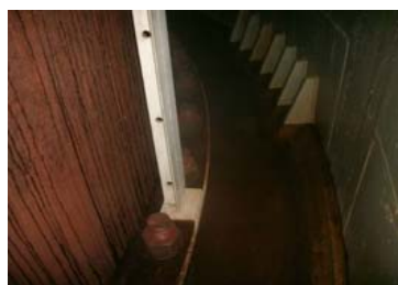
RPV support skirt •No external equipment abnormality though some rust on foundation bolts.
