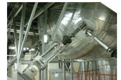
Moisture separator •No external equipment abnormality
