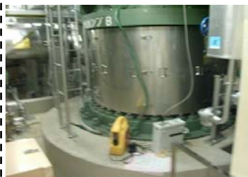
RHR pump •No external equipment abnormality
