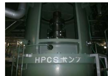
HPCS pump •No external equipment abnormality
