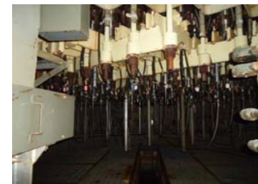
In pedestal •No external equipment abnormality
