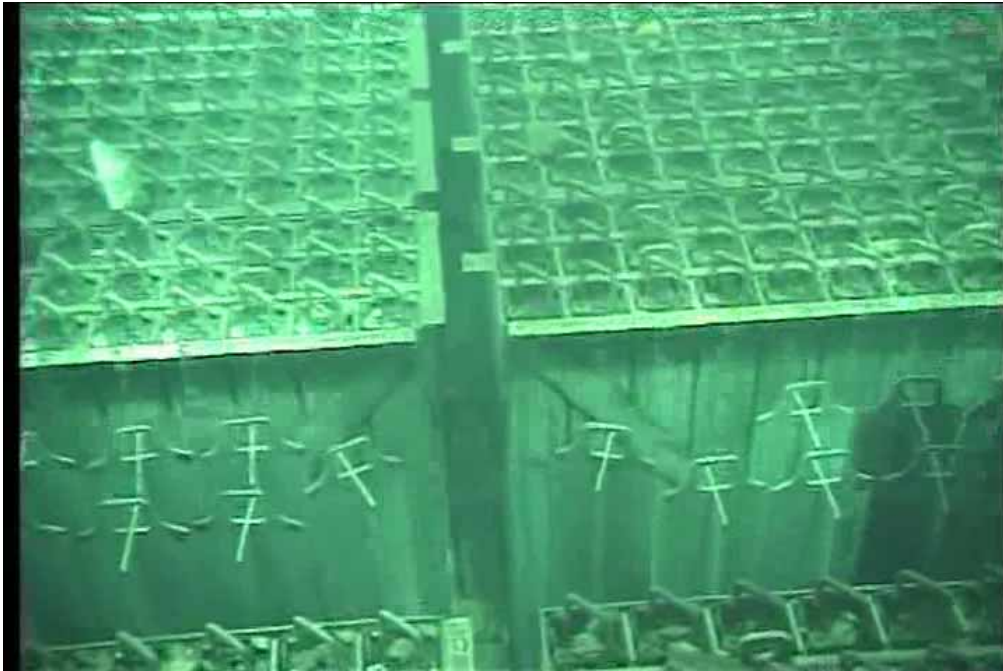
Figure 8 Conditions within Unit 4 SFP (3)
