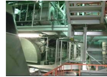
EDG 6A •No external equipment abnormality •Standby
