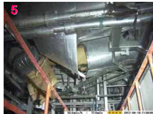
5 Northeast corridor upper area
