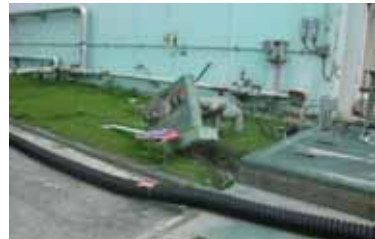
⑬ Unit 4 water sampling outlet removal from foundation of sampling outlet (presumed to be tsunami impact)
