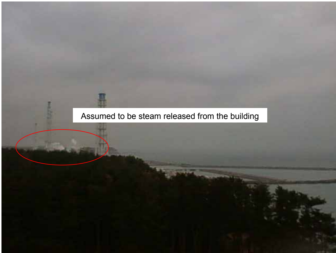
Fukuichi Live Camera footage (Around 10:00, March 15)
