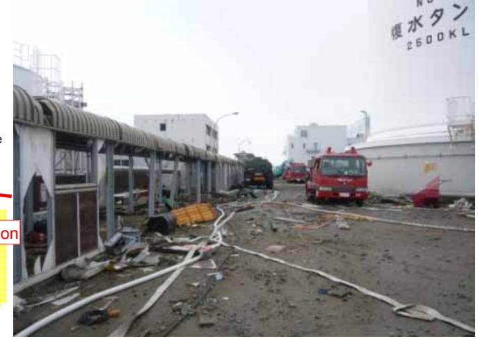
No particular abnormality with the road but scattered rubble. Photo taken 3/16
