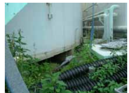
⑧ Unit 2 Condensate storage tank lower area • Ground under tank collapsed. No leakage
