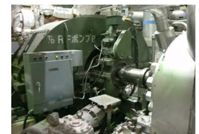
Turbine-driven reactor feedwater pump •No external equipment abnormality
