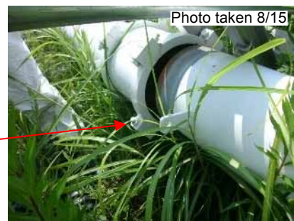
• Support for another pipe at a joint for the transformer disaster prevention pipe (filtered water tank source) became slanted due to collapse of the slope. Said joint made contact and caused leakage.
