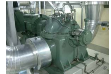
Turbine component cooling pump •No external equipment abnormality
