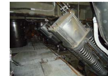
MSIV •No external equipment abnormality
