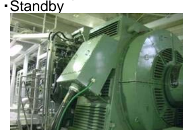
EDG (HPCS) •No external equipment abnormality
