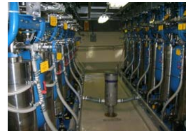
Hydraulic control unit •No external equipment abnormality
