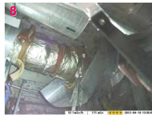
8 Southeast S/C manway upper area
