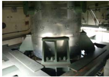
RHR heat exchanger •No external equipment abnormality
