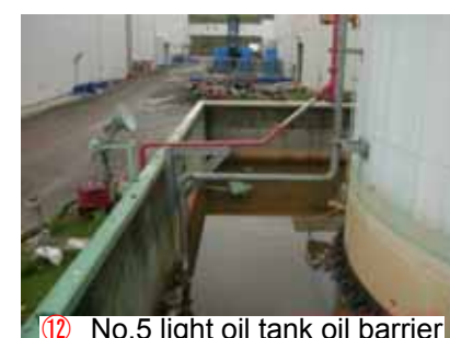
⑫ No.5 light oil tank oil barrier
