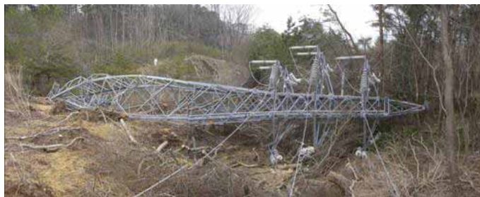
Figure 2. Yorunomori Line No. 27 transmission tower
