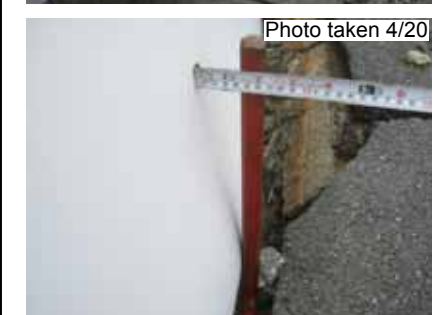
• Deformation due to collapse of tank lower area
