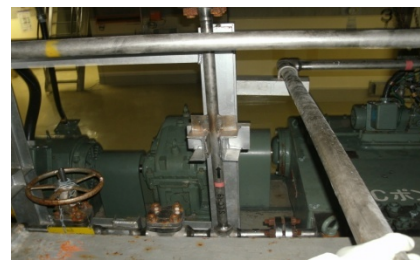
SLCS pump •No external equipment abnormality
