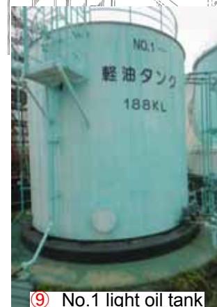
⑨ No.1 light oil tank
