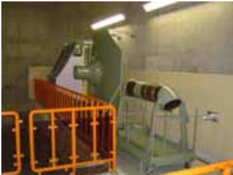
New reinforcements installed
