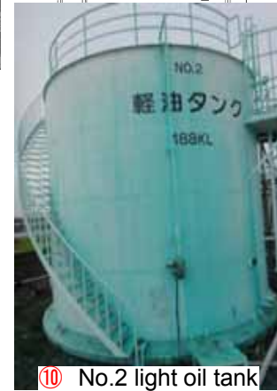
⑩ No.2 light oil tank
