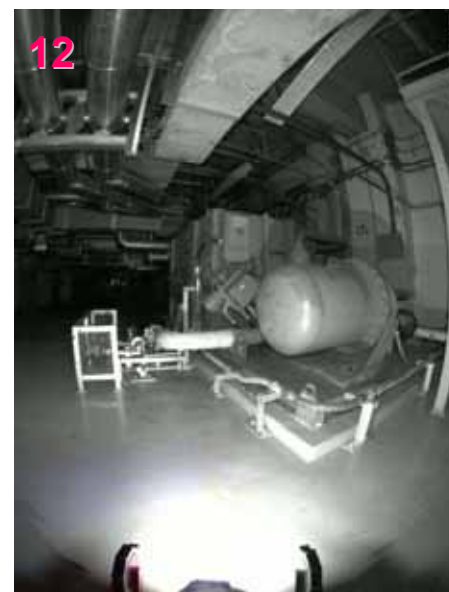
Flammability control system -No external equipment damage found
