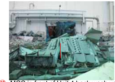
⑬ MCC in front of Unit 4 back wash valve • MCC collapsed
