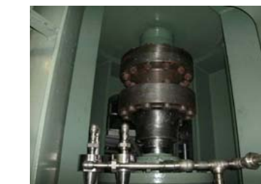
Low pressure condensate pump •No external equipment abnormality
