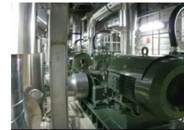
Reactor component cooling pump No external equipment abnormality
