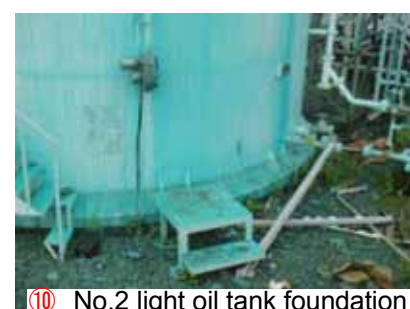
⑩ No.2 light oil tank foundation
