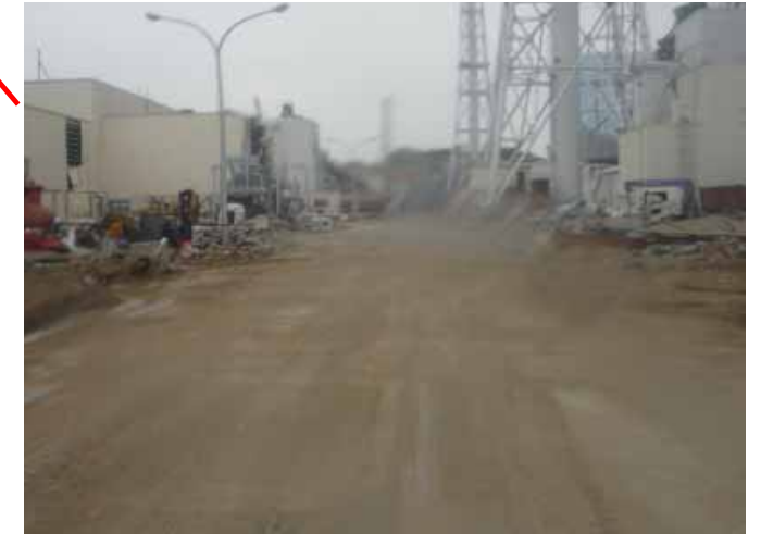
No particular abnormality with Units 1 to 4 west side road. Rubble was scattered when Units 1, 3, 4 R/B were damaged. Photo taken 3/20
