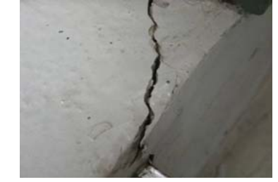
Feedwater heater •There is slight cracking on the fixed leg foundation for feedwater heater 5B but there is no other external equipment damage.
