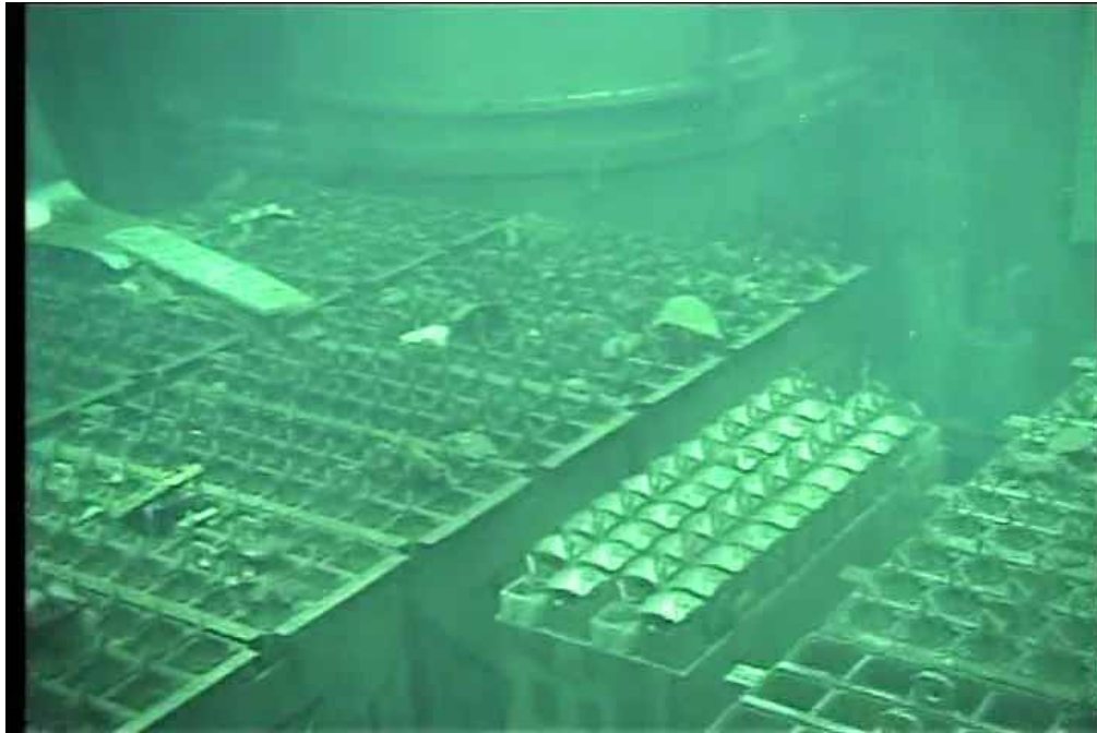
Figure 6 Conditions within Unit 4 SFP (1)
