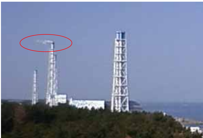
Faint steam-like mass seen toward mountain side of Units 3/4 exhaust stack
