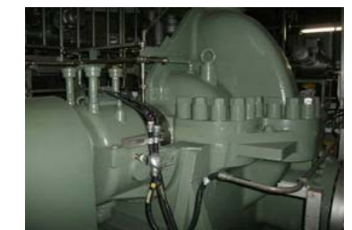
High pressure condensate pump •No external equipment abnormality
