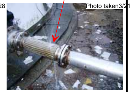
• Leakage after earthquake, tank outlet root valve open.
