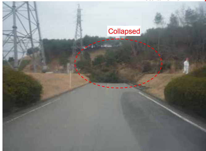
Though not a priority emergency route, the slope failed and the road was blocked and impassable. Photo taken 3/20
