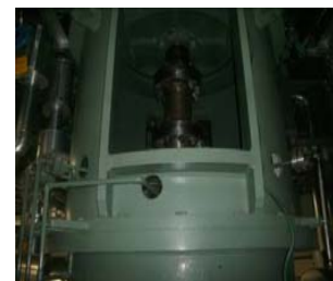
LPCI pump •No external equipment abnormality
