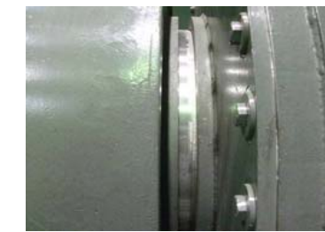
Low pressure turbine •Sliding marks on No.3 bearing high pressure side rotor •Sliding marks on No.3, No.8 bearing rotor •Sliding marks on No.8 bearing generator side rotor
