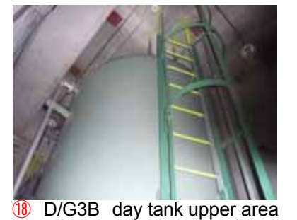
⑱ D/G3B day tank upper area
