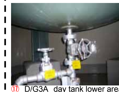
⑰ D/G3A day tank lower area
