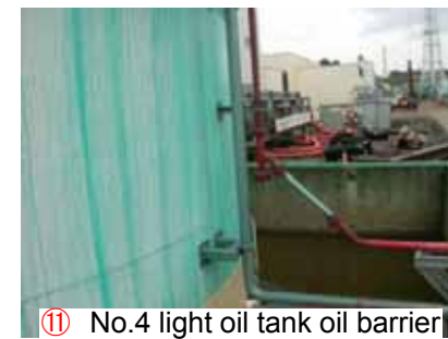
⑪ No.4 light oil tank oil barrier
