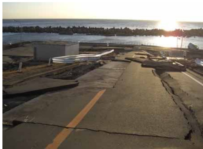
Reinforcement work was conducted on this road, but cracks and subsidence was found on both sides of the road which were not reinforced. Photo taken 3/17
