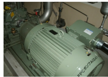
Fuel pool cooling & clean up pump •No external equipment abnormality
