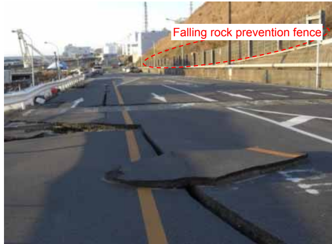
One side of the road on the seaside was cracked and subsided in parallel with road. West side was accessible. Photo taken 3/17
