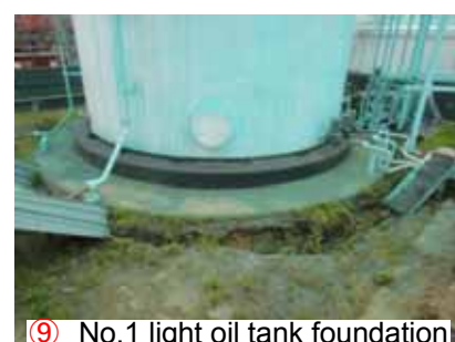
⑨ No.1 light oil tank foundation
