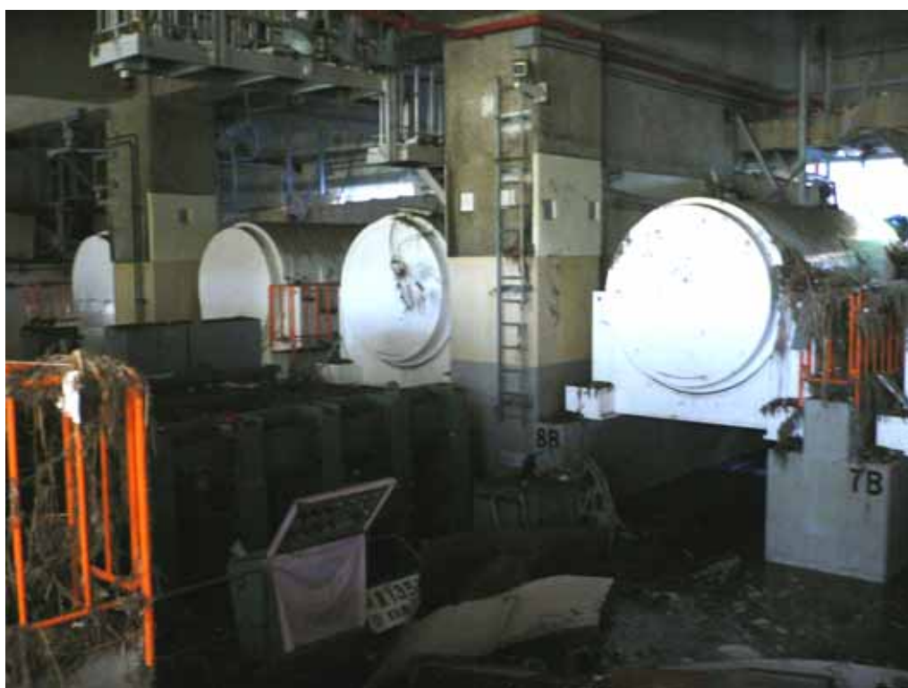
Figure 3 Conditions inside the dry storage cask storage building
