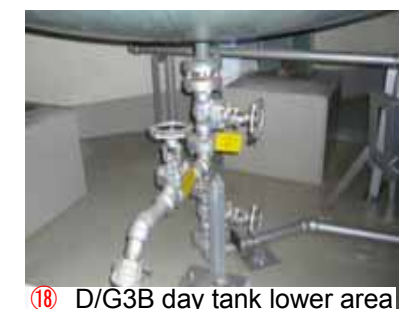
⑱ D/G3B day tank lower area
