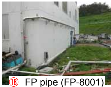
⑮ FP pipe/building interface • No major external damage to pipes in trench
