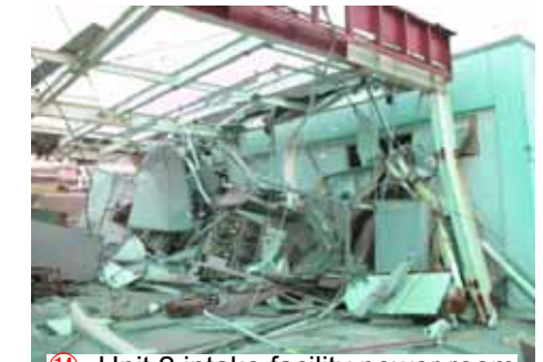
⑭ Unit 2 intake facility power room • Unit 2 power room collapsed
