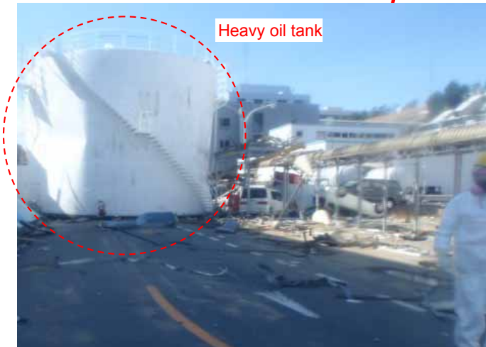
No major damage to the road, but the heavy oil tank carried by the tsunami blocked the road making it impassable. Photo taken 3/17
