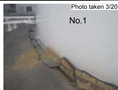
• Deformation due to collapse of tank lower area
