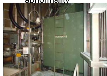
Reactor recirculation pump •No external equipment abnormality though some rust on mount bolts and nuts.
