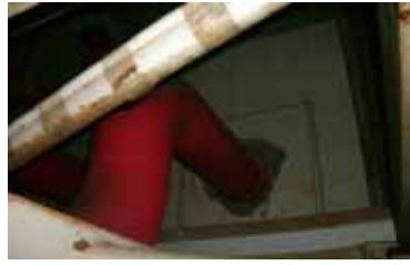
⑮ FP pipe/building interface • No major external damage to pipes in trench
