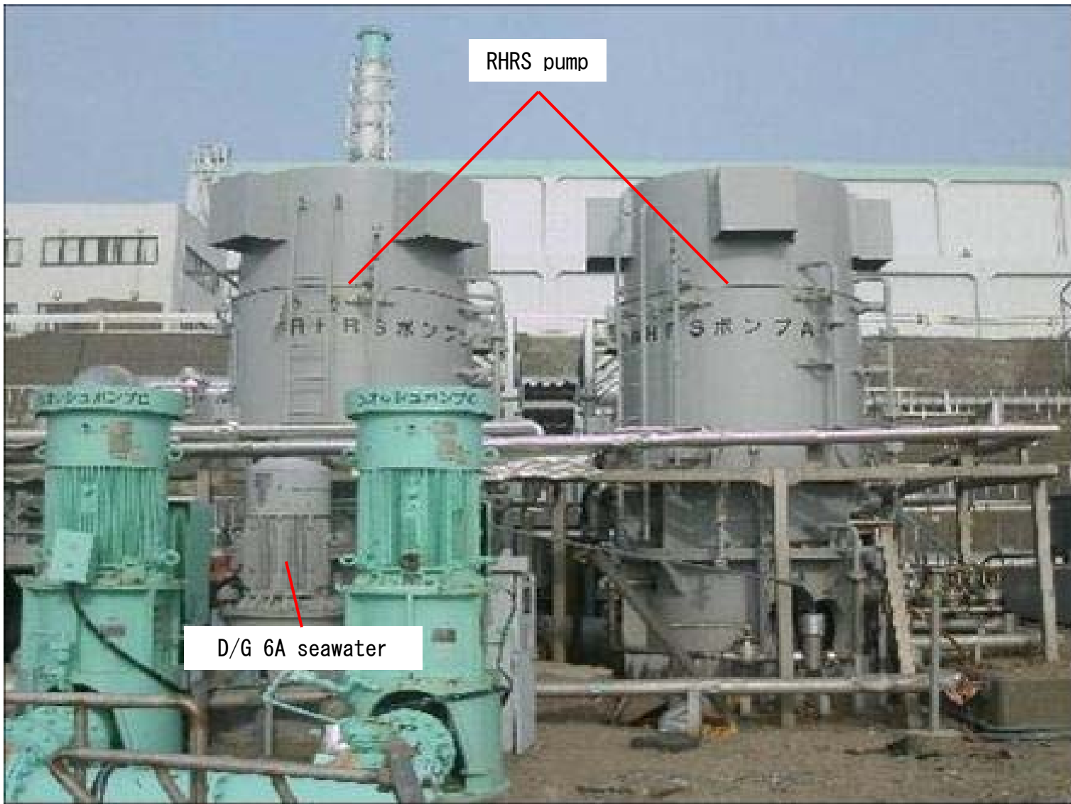
Fukushima Daiichi Unit 6 state of emergency seawater
