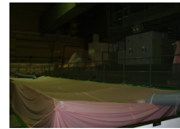
SPF •No external equipment abnormality (covered for condensation)
