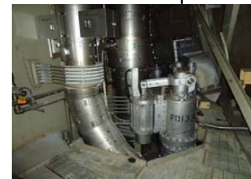
SRV •No external equipment abnormality
