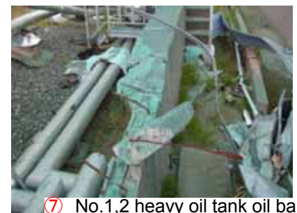
⑦ No.1,2 heavy oil tank oil barrier • Found cracks in oil barrier
