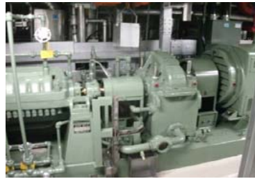
CRD pump •No external equipment abnormality
