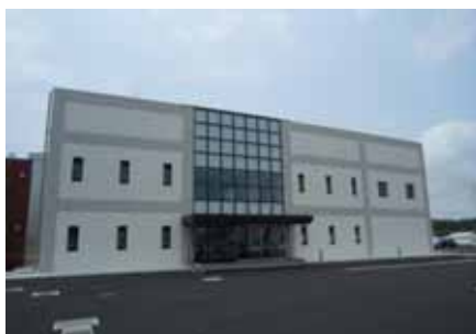
Outer view of seismic isolated building
