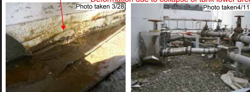
• Leakage from bottom of tank
