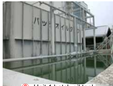
⑥ Unit 1 batch oil tank • No major external abnormalities including oil barrier
