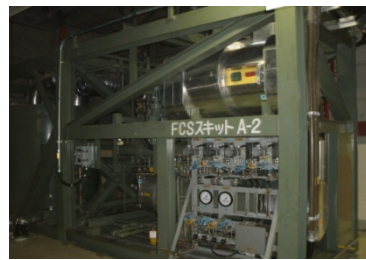
Flammability control system •Subsystem A has no external equipment abnormality •Subsystem B (installed on 3F) has had defect in cooler in B-2 recombiner since before earthquake
