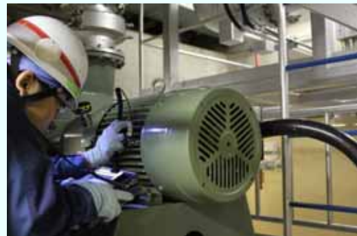
Vibration measurement being performed on the electric motor of the emergency gas treatment system (A) [Permanent installation completed on December 14, 2012] (Photo taken on December 14, 2012)
