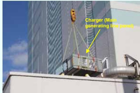
Charger (Main generating line panel) being carried in (Photo taken on November 21, 2012)
