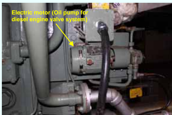
Electric motor installation (Oil pump for diesel engine valve system*2) (Photo taken on December 14, 2012)
