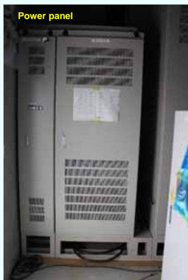
Installation of power panel of Units 1-2 discharge channel monitor (Photo taken on December 18, 2012)
