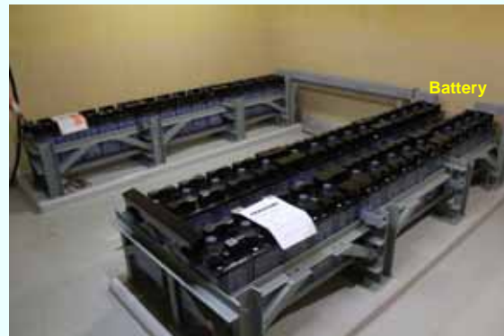
Battery installation [Installation completed on December 18, 2012] (Photo taken on December 25, 2012)
