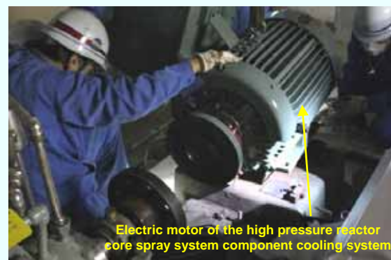
Electric motor installation [Completed on December 13, 2012] (Photo taken on December 13, 2012)
