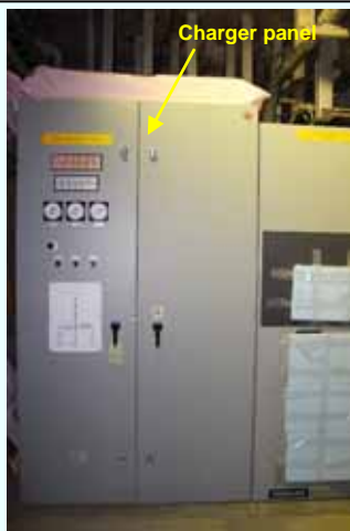
Charger panel installation [Installation completed on December 3, 2012] (Photo taken on December 25, 2012)
