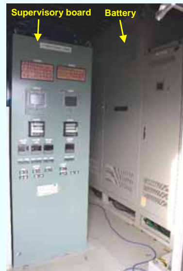
Installation of supervisory board, etc. of Units 1-2 discharge channel monitor [Installation completed on December 10, 2012] (Photo taken on December 18, 2012)
