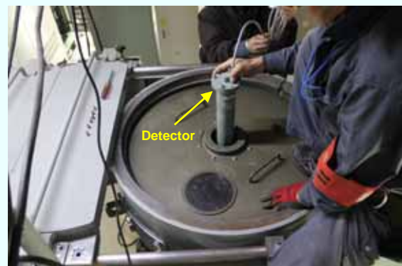
Units 1-2 discharge channel monitor (detector) installation (Photo taken on December 18, 2012)
