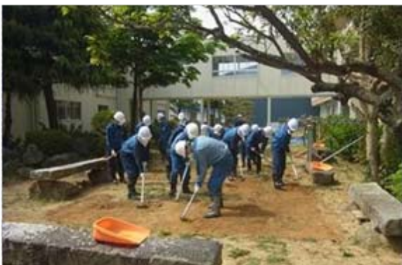
[Simple decontamination work in school facilities]
