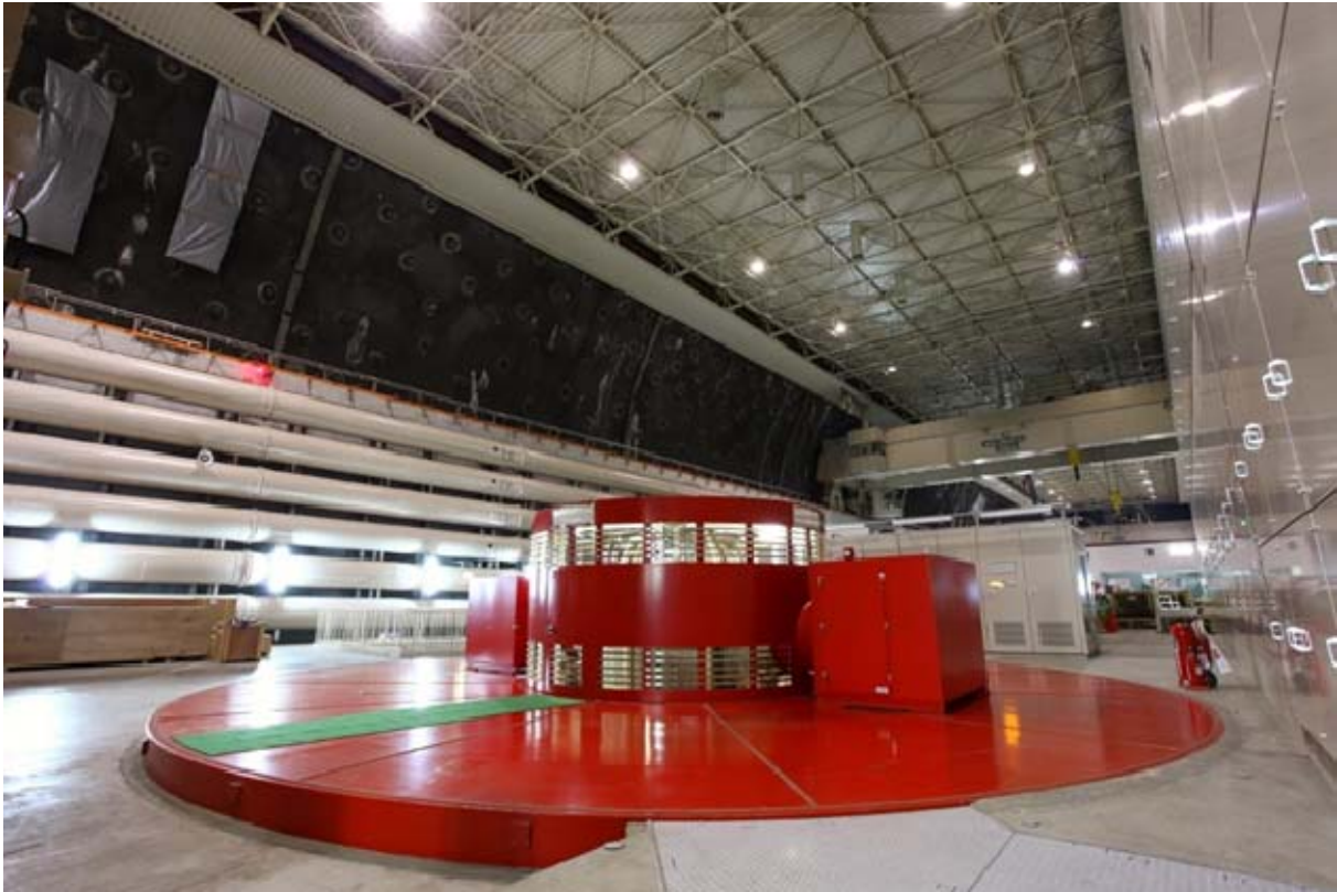
※Foreground: Unit 4 (started operation today)
