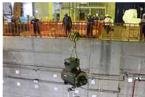
Motor replacement (transporting spare motors)
