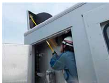
Training on the manual opening/closing of power truck intake/exhaust dampers in the event of a malfunction
