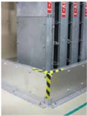
Surrounding building the floor penetration seals with sheet metal dikes
