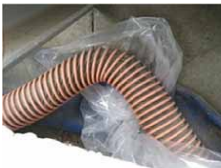
Hose used for water transfer
