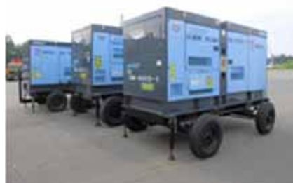
Fitting engine generators with wheels (Kashiwazaki-Kariwa)
