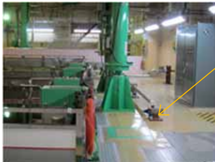
Installation of spray piping from the outside of the building to the spent fuel pools (Unit 2)
