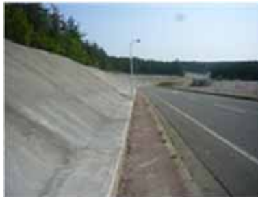
Creation of fire belt at the power station site
