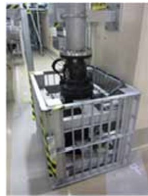
Permanent drainage pump in the residual heat removal system pump room (Unit 7)
