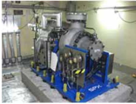
Installation of the alternate high-pressure coolant injection system pump
