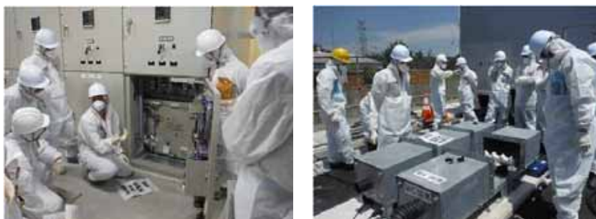
Training on laying and connecting high-voltage cables (Fukushima Daiichi)
