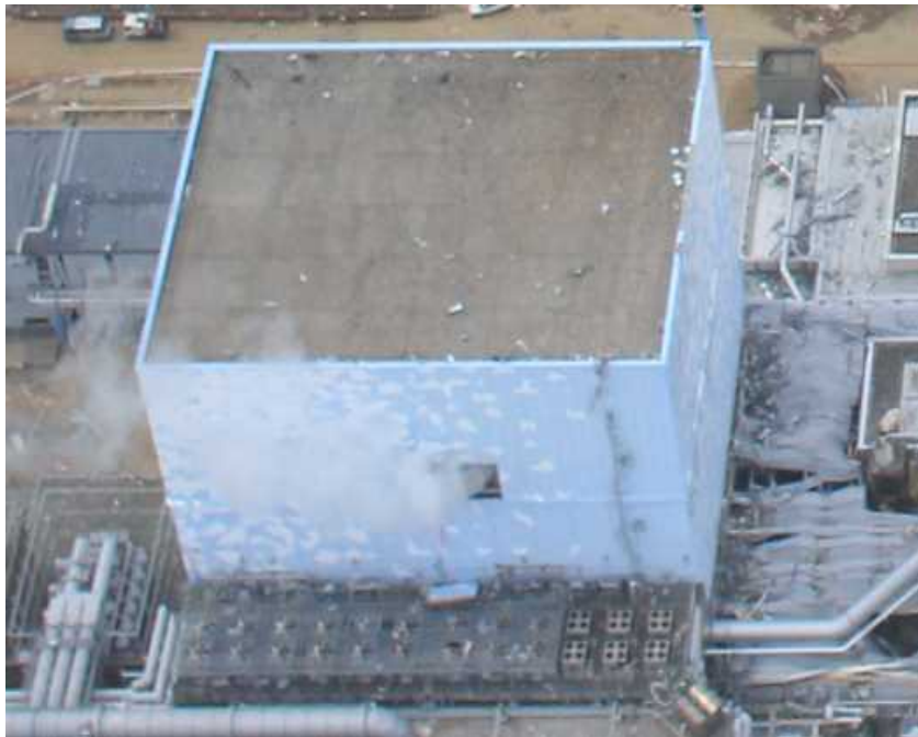
Figure Opened blow-out panel of Unit-2
