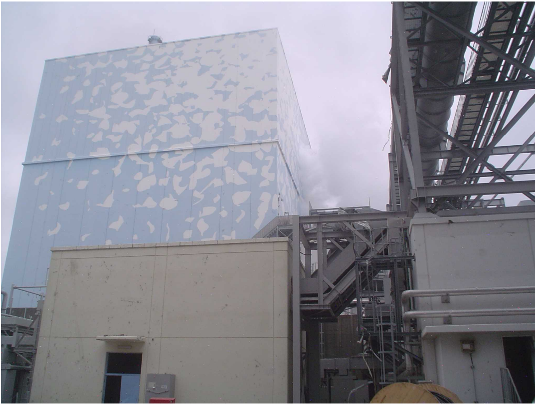
Figure 9 Steam release from Unit-2 (taken at 08:58 on March 15 th )
