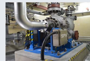
Alternate high-pressure cooling water injection system pump at Unit 7 (Installed system)
