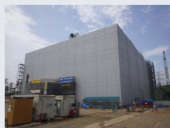
Exterior of miscellaneous waste incinerator
