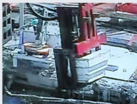
Removal of large piece of rubble from SFP at Unit 3
