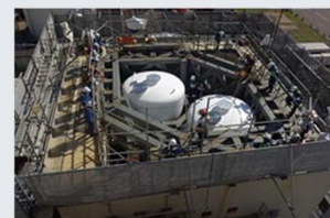
Above-ground filtered venting system at Unit 7 (Fitted with iodine filters)
