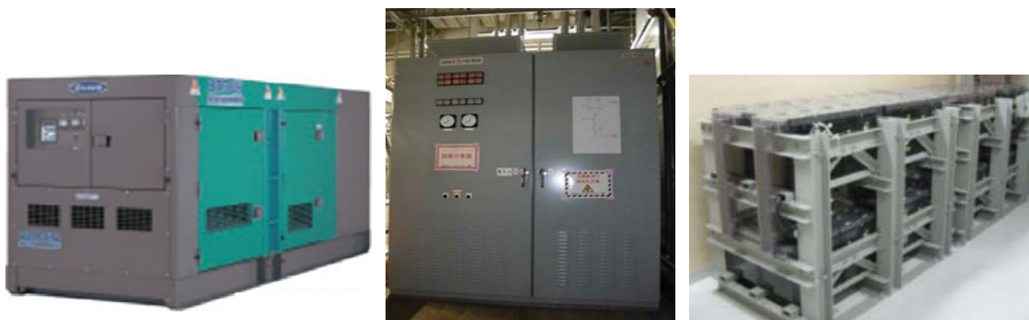
Alternate DC power sources (Left: recharging generator, Center: recharging panel, Right: storage batteries)
