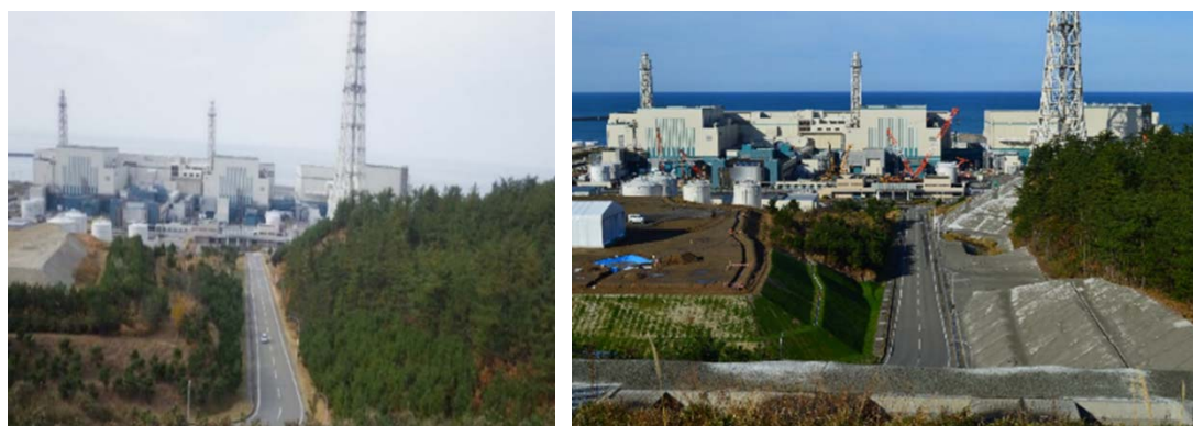
Power station facility firebreak (Unit 5-7 side) (Left: prior to construction, Right: after construction)
