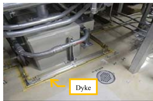
Dyke (to prevent oil leaks from spreading)
