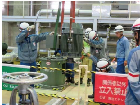
In-house engineers replacing electric motor for vertical pump generators
