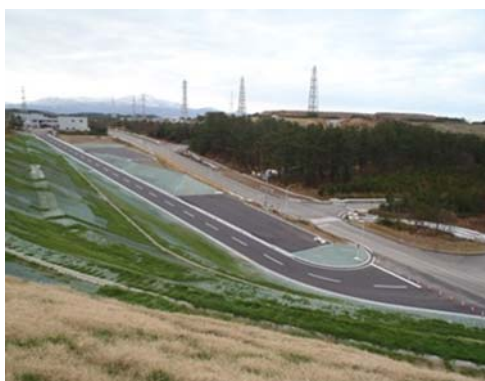
Access routes additionally built on the mountain side of Units 5-7
