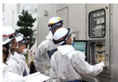
Adjusting voltage and frequency after starting up the power supply truck
