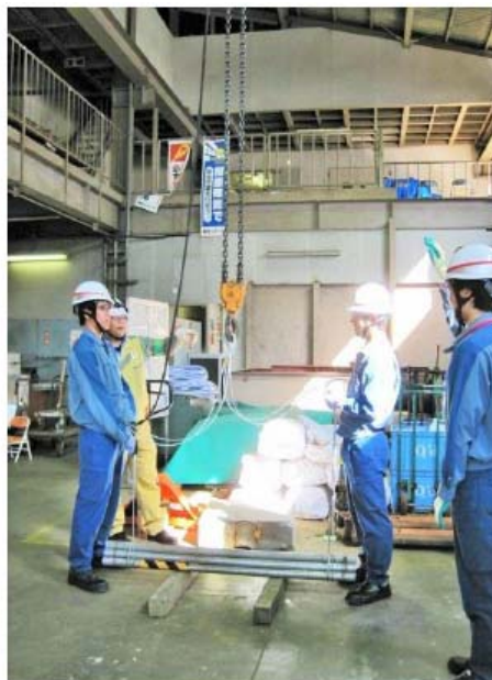
Hoisting of heavy materials
