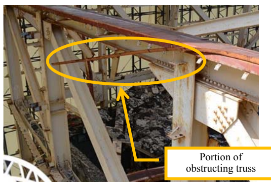
Conditions on the 5 th floor of the Unit 1 reactor building (locating trusses that will hinder dismantling work)
