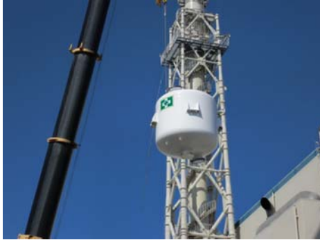
Iodine filter installation (Unit 7)
