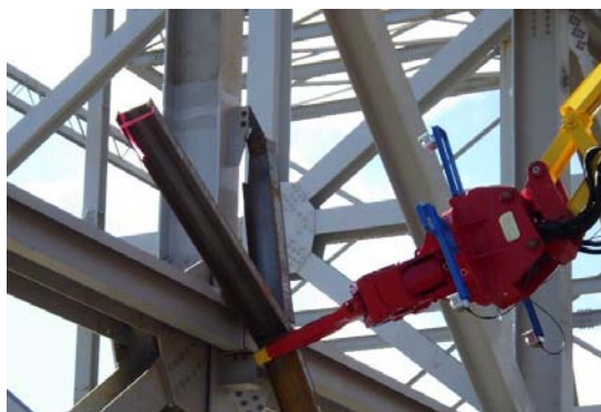
Training facility built in Hirono Town to train personnel on using equipment for removing obstructing steel trusses (began on December 3)
