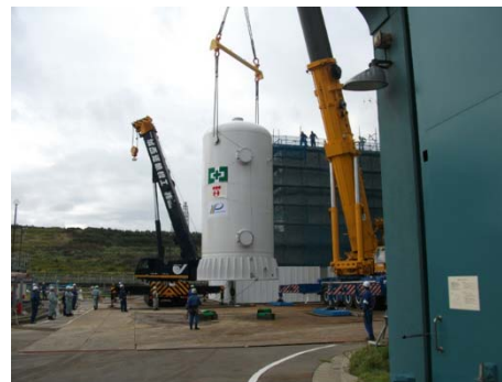
Robot used to survey the opening of the reactor containment vessel Installation of filtered venting equipment (Kashiwazaki-Kariwa Unit 7)
