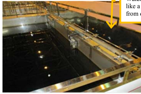
Spent fuel pool external spray equipment
