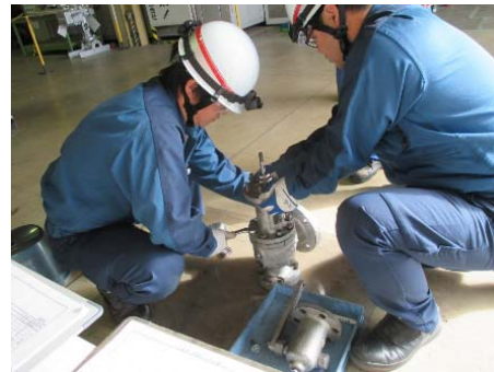
In-house engineers disassembling and inspecting safety relief valves
