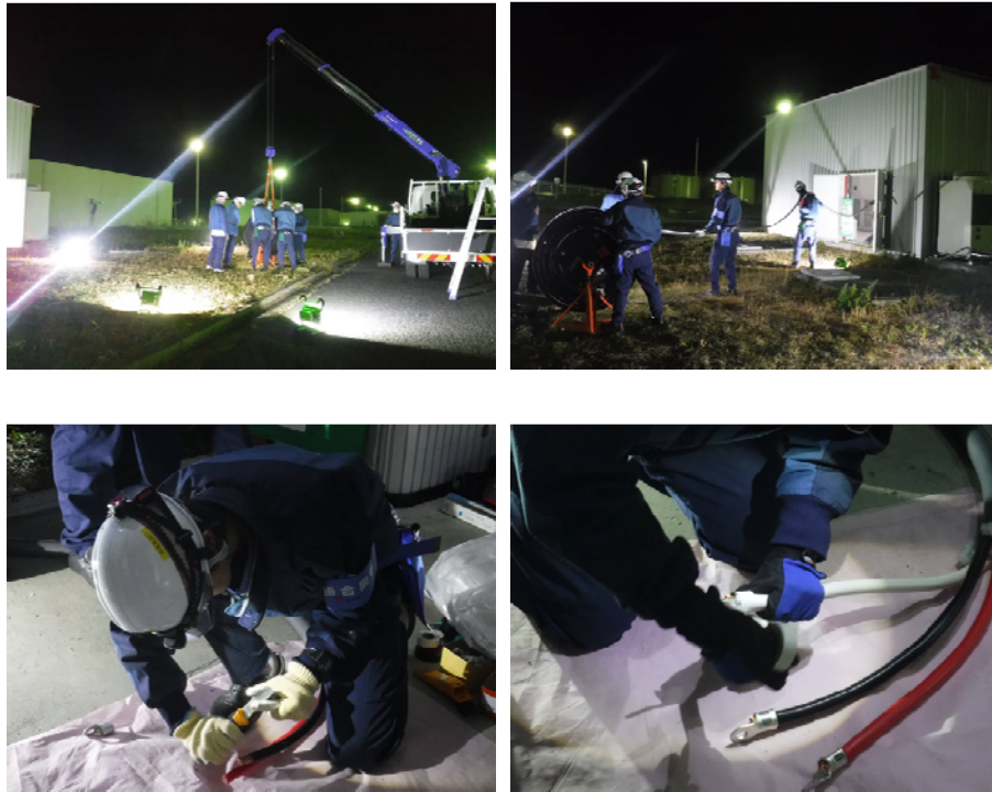
Night training on laying and connecting cables (Fukushima Daini)
