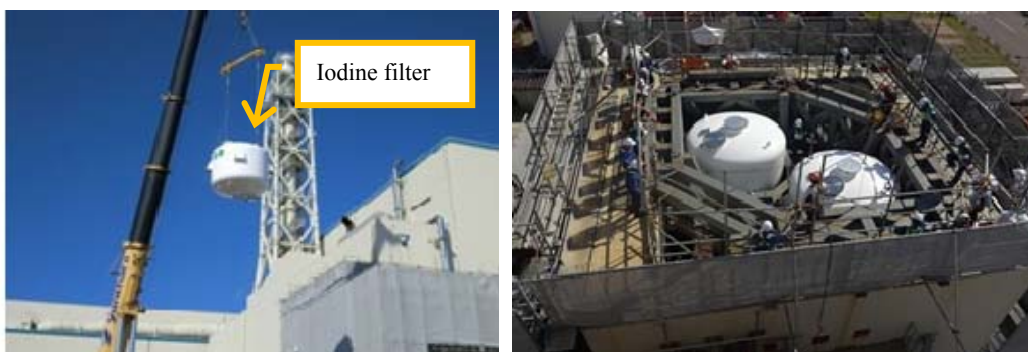
Above-ground filter venting equipment installation (Unit 7)
