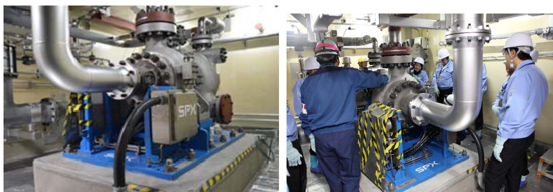
High-pressure alternate coolant injection system pump installation (Unit 7) (work is being observed by Nuclear Reform Monitoring Committee members (right))
