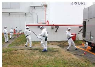
Pulling cables out of power supply trucks
