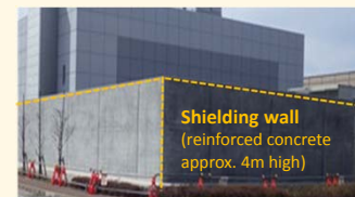
Shielding installed around the main base-isolated building to protect responders from exposure
