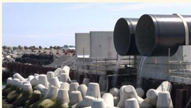
Drainage channel K outlet switched to inside port
