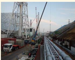
Freezing pipes on the west side of Units 2-4
