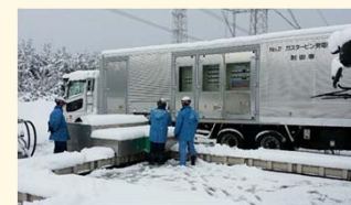
Training in operating a gas-turbine generating vehicle in a snowy environment
