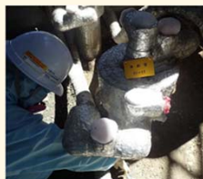
Freezing initiated of land-side impermeable wall
