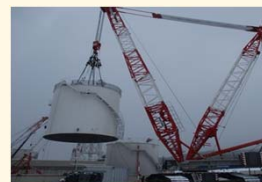
Replacement with thick steel-panel light oil tanks capable of withstand collisions with flying rubble
