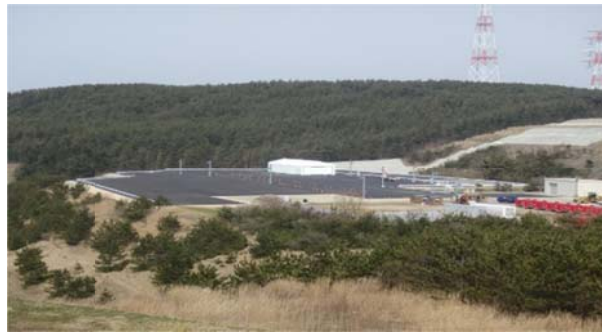
Elevated parking area constructed on the Ominato side (paved area)
