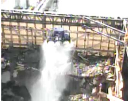
Spraying anti-scattering agent on rubble
