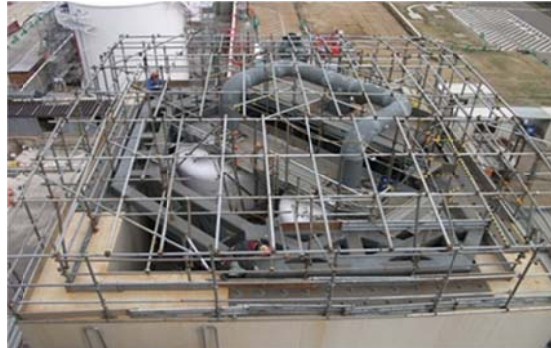
Pipes fitted around an iodine filter (Unit 7)
