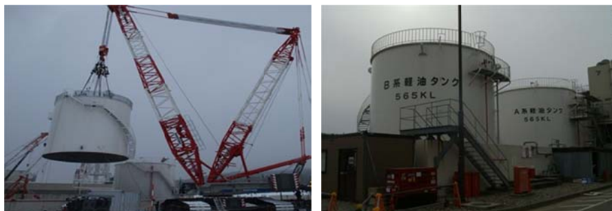
Replacing light oil tanks (Unit 7) (left: tank being lifted; right rear: installed tanks)
