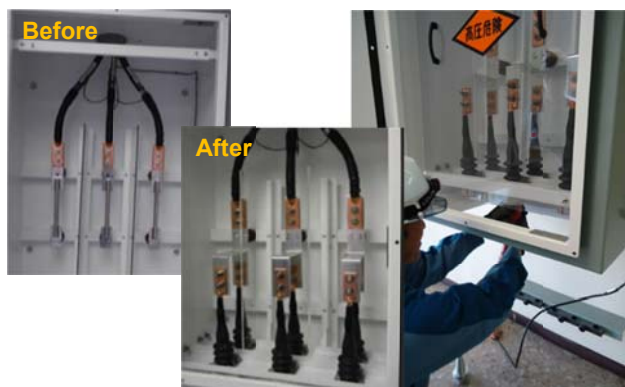
Improved power cable connection terminals from power supply cars (Fukushima Daini NPS)
