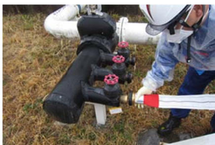
Ensuring a means for fire engines to inject cooling water (Fukushima Daiichi NPS)
