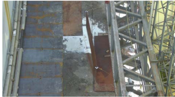
Steel plates fitted for installation of pipes extending to spray nozzles
