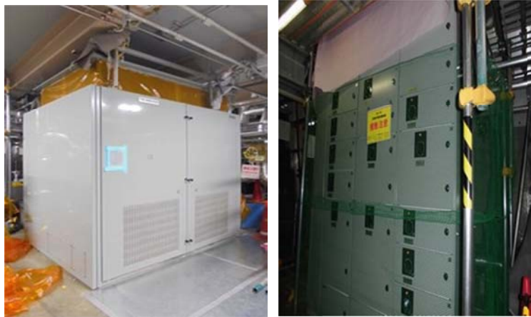
Transformer and switchboard added for station electrical system (Unit 7)
