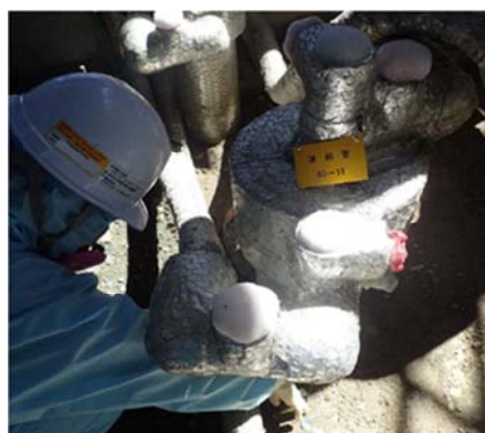
Freezing pipes (west side of buildings at Units 2-4) Conditions after freezing initiated
