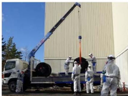
Signaler issuing cues to load a cable reel
