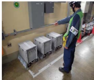
High-performance lithium batteries deployed in control zones (Kashiwazaki-Kariwa NPS)
