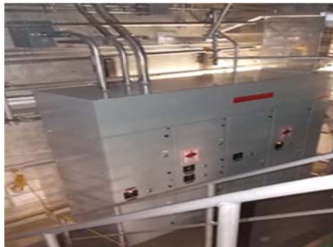
DC125V switchboard for alternate high-pressure cooling water injection system pump (Unit 7)
