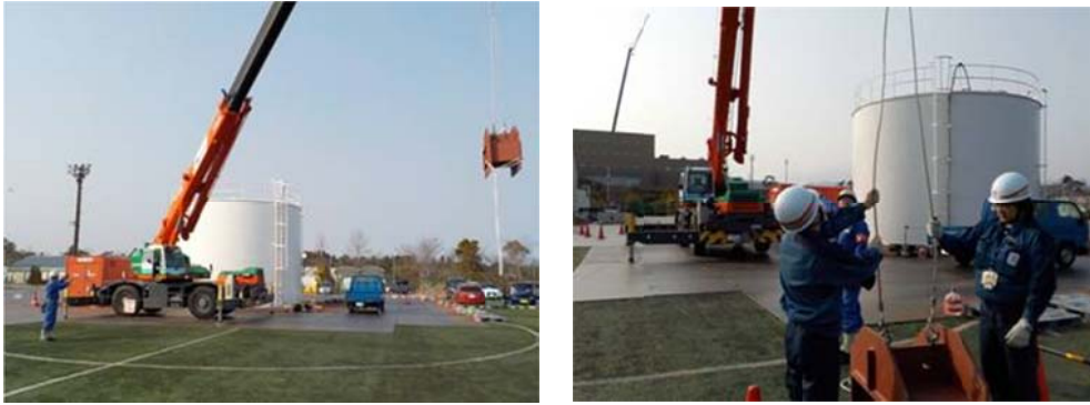
Training in mobile crane operation (Fukushima Daiichi NPS (training conducted in J-Village))
