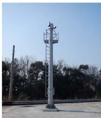
Detector installed at elevated parking area
