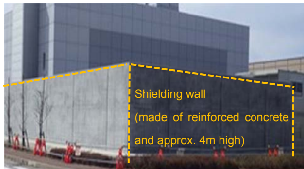
Shielding wall around main base-isolated building
