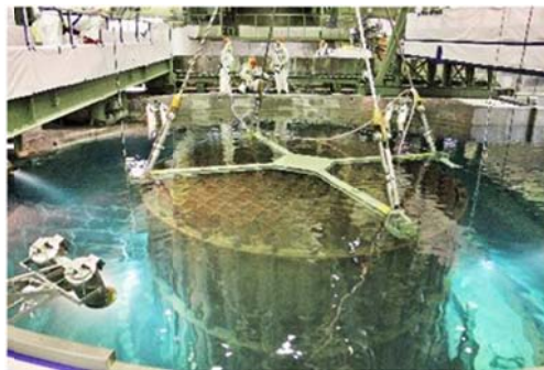
Work of moving steam-water separator into reactor
