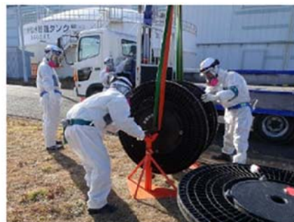
Unloading a cable reel
