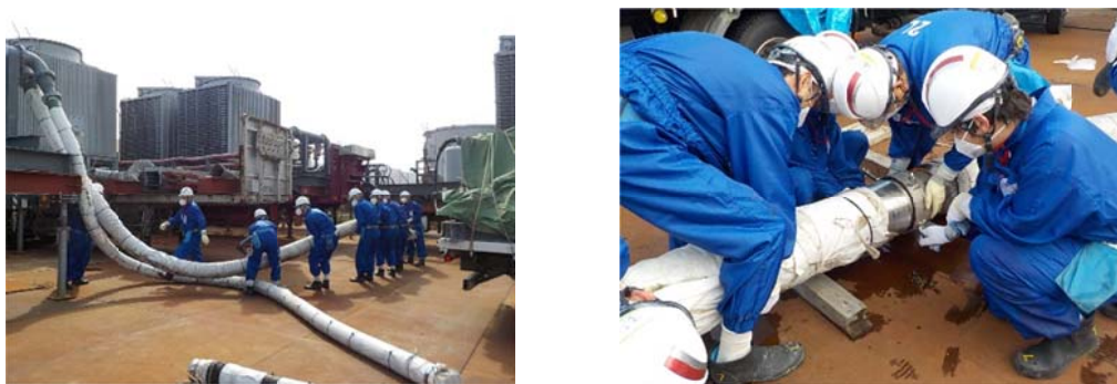
Training on connecting spent fuel pool cooling water injection equipment (Fukushima Daiichi) (The photo on the left shows the air cooling unit)
