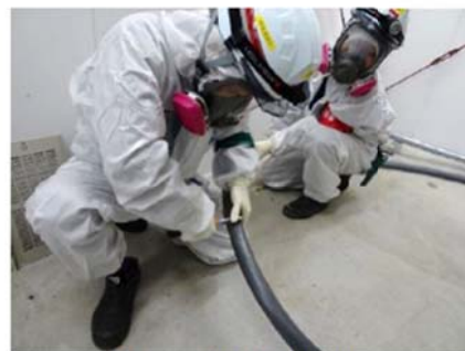
Splicing a cable
