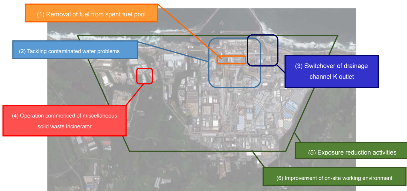
Progress made on the principal work at Fukushima Daiichi NPS
