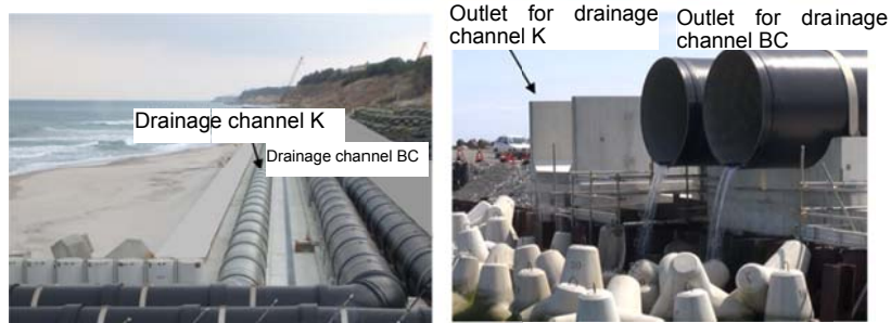
Outlet for drainage channel K after switchover
