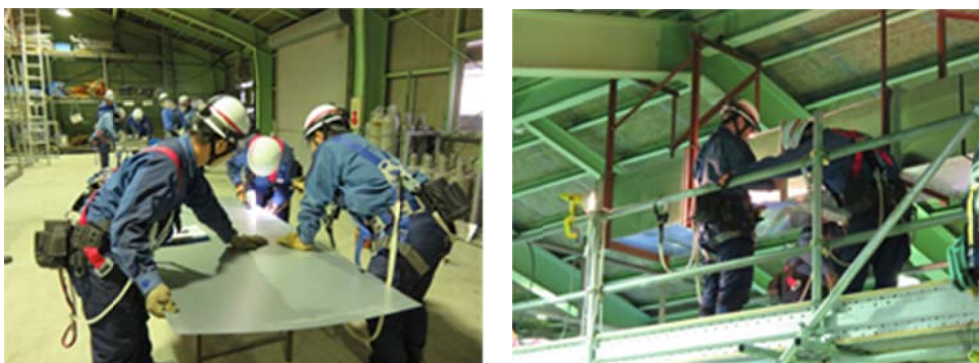
Training in repairing ventilation system ducts (Kashiwazaki-Kariwa NPS) (Left: material processing; right: repairing a duct at a high height)
