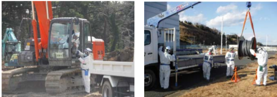
Training in removing rubble and connecting temporary cables while wearing full-face masks (Fukushima Daini NPS)
