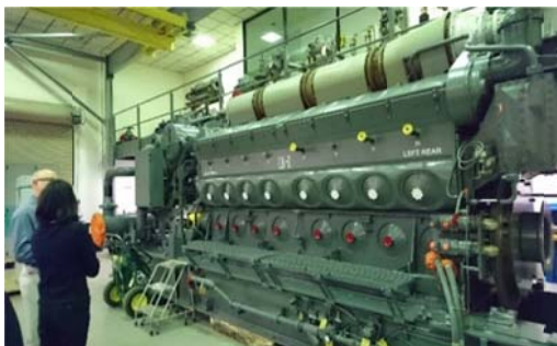
Inspection of training facility (diesel generator)
