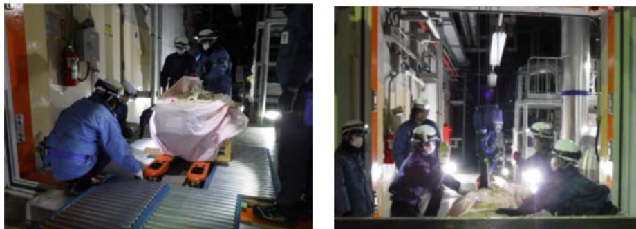
Training in replacing electric motors at night (Fukushima Daini NPS)
